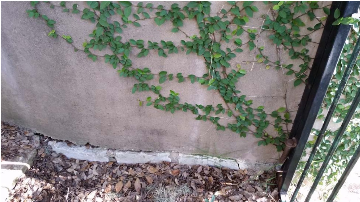
Fig. 5. Pool deck wall bearing on masonry.
