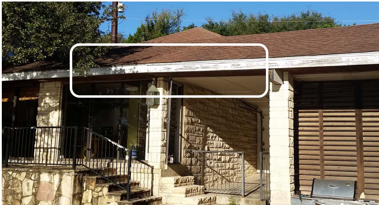
Fig. 1. Bowing of roofline at rear of house.
