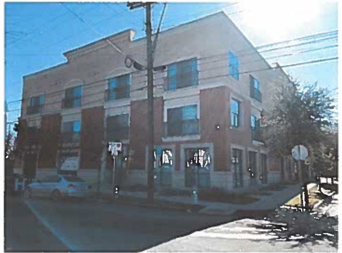
1401 E. 4TH ST. (MULTIFAMILY)
