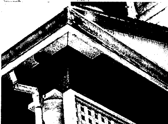
Damaged exterior wall materials can be repaired or replaced in-kind, as in the fascia board to the left.
