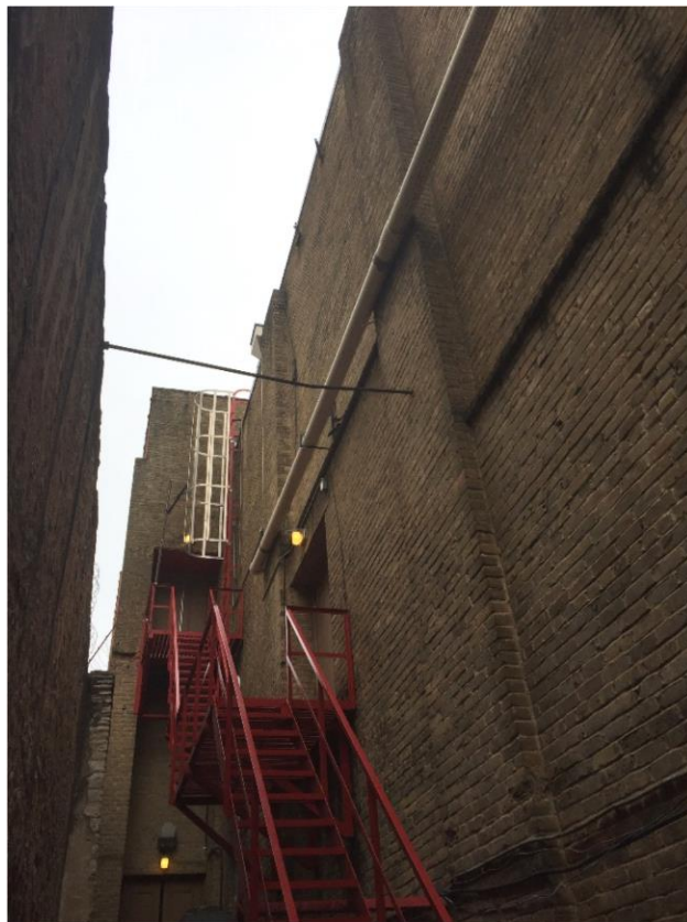
These fire escapes increase the cost and expertise necessary to construct scaffolding from the ground to the top of the building
