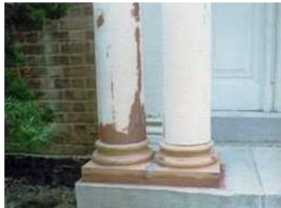
Deteriorated wood porch elements can be repaired in place with epoxy consolidants and fillers.
