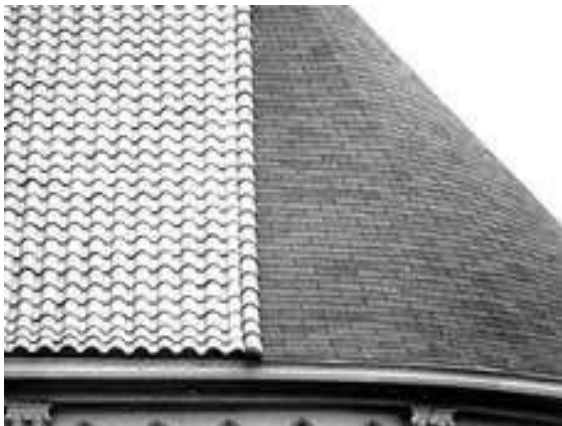
Asphalt shingles are an incompatible replacement substitute for the original Spanish clay tiles.
