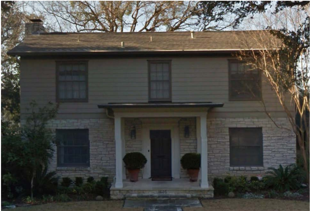
2014 photograph of the house showing the stone veneer
