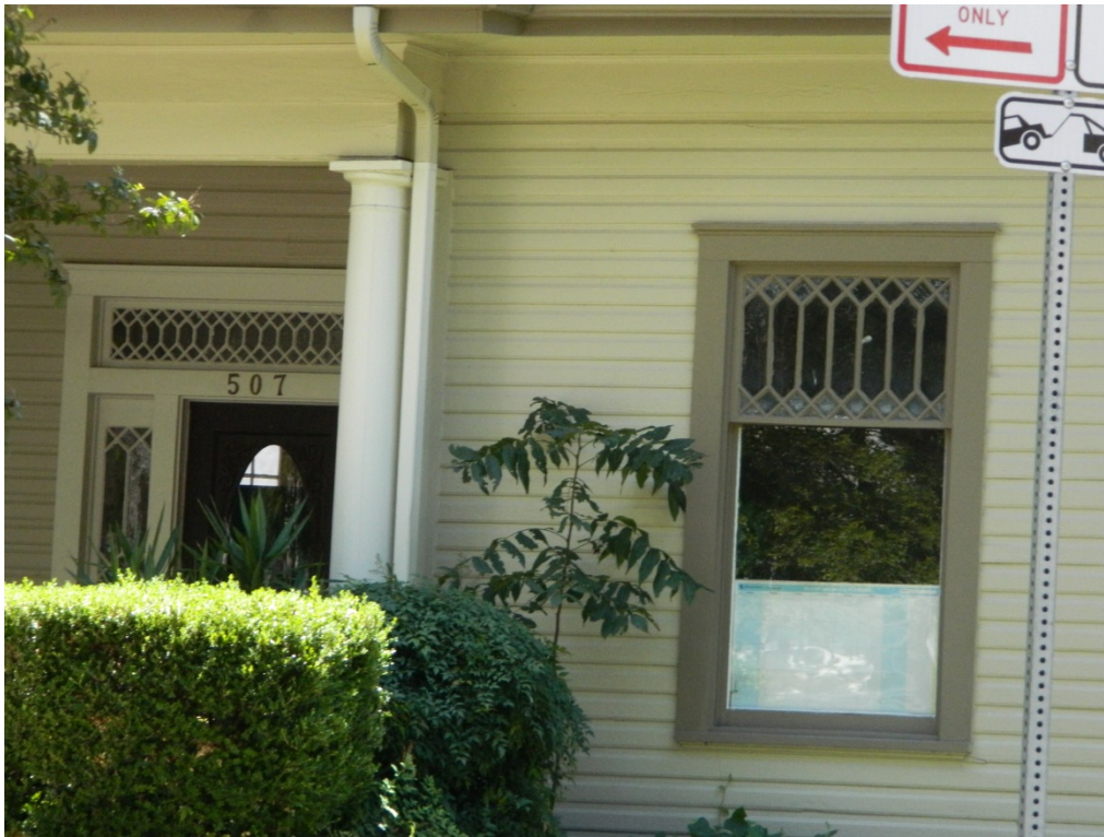
Detail of decorative upper sashes in the front windows, the sidelights, and transom
