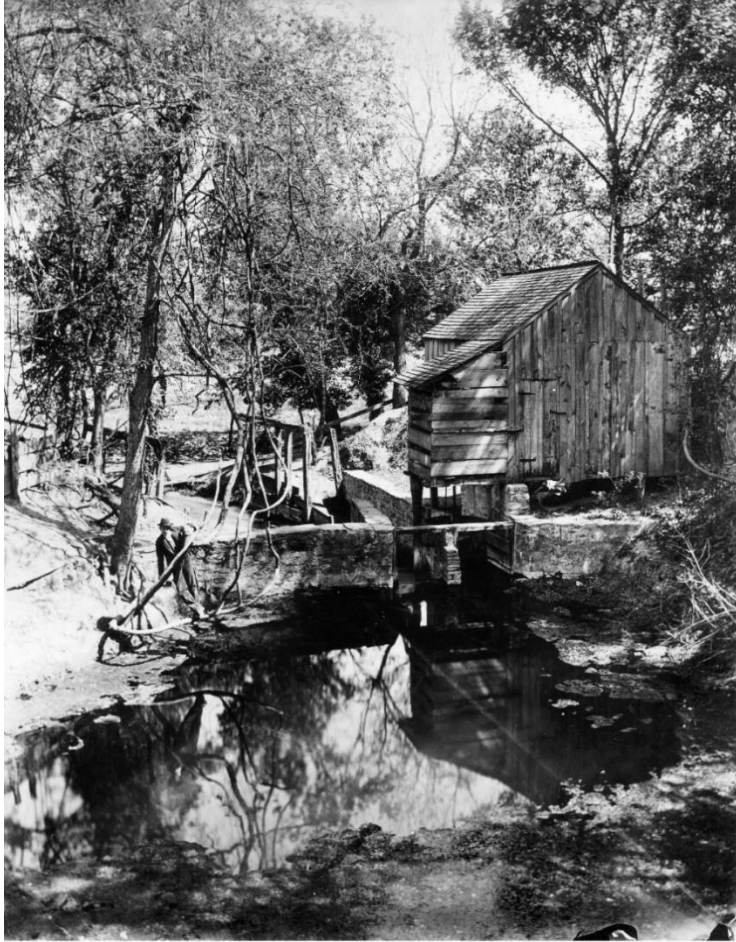
Figure 10. Photo of the Old Mill Spring and Paggi's Mill circa 1876. This is the earliest known photo of Old Mill Spring. The wall impounded the spring pool, slowing down the water velocity and increasing the water depth. Today most of the rock wall from the 1800s is gone. Photo from Austin History Center, C03293.
