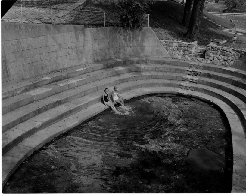
Figure 6. Eliza Spring in 1953. The spring flow was buried into a pipe underneath the lawn of Barton Springs and the amphitheater keyway filled in with masonry. A chain link fence was also added to the top of the amphitheater. The natural substrate in the spring pool can be seen. Photo from the Austin History Center.
