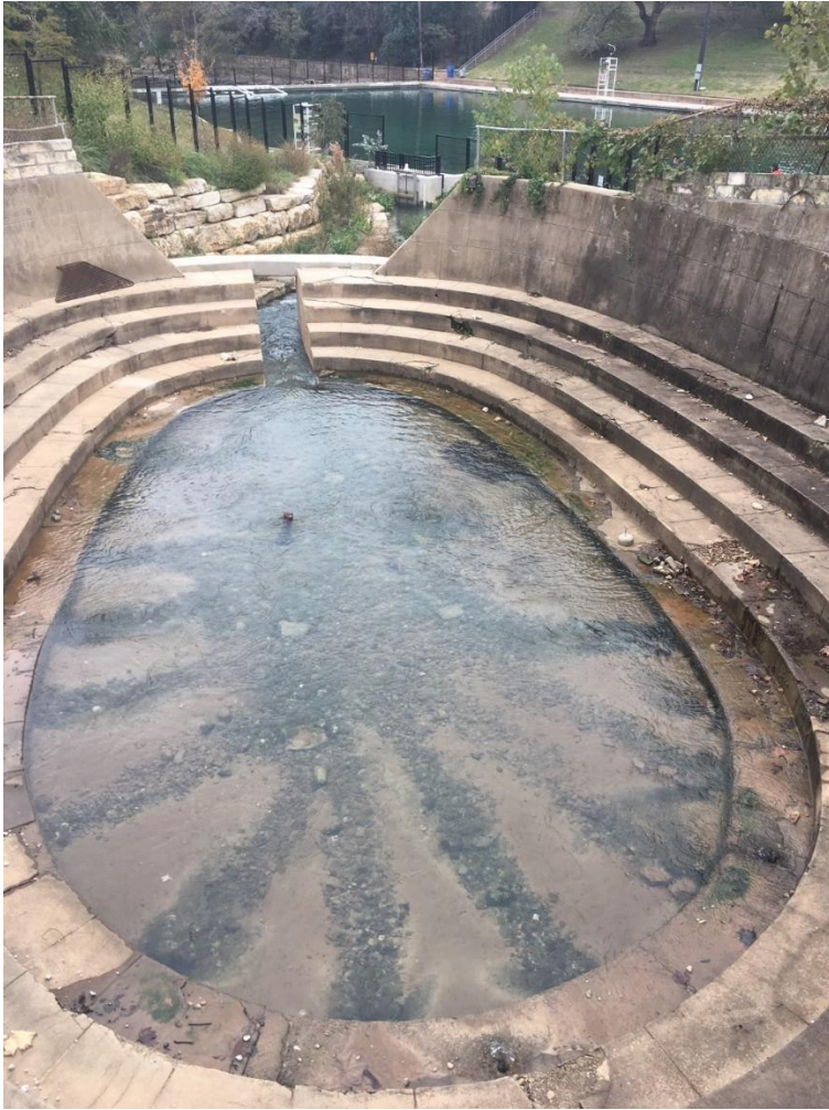
Figure 8. Eliza Spring in November 2018. The surface stream is reestablished and masonry removed from the keyway. The floor of the spring pool is covered in concrete, with limestone gravel added on top for salamander habitat. Lines of gravel substrate connecting the edge of the spring pool to the center follow the path of water leaving spring outlets along the concrete steps.
