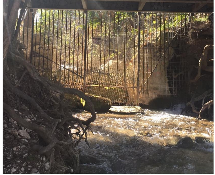
Figure 13. Waterfall installed at the Old Mill stream near Barton Creek in 2004 (left) and in 2019 (right) with the barrier fence installed. Concrete was removed from the water after construction. In the right, water is bypassing the waterfall and exiting through a cavity on the right bank near Barton Creek.
