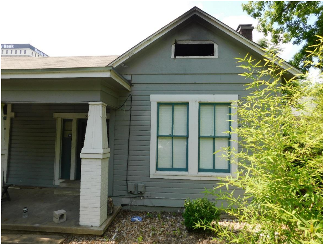
Detail of the front of the house showing fire damage to the attic vent
