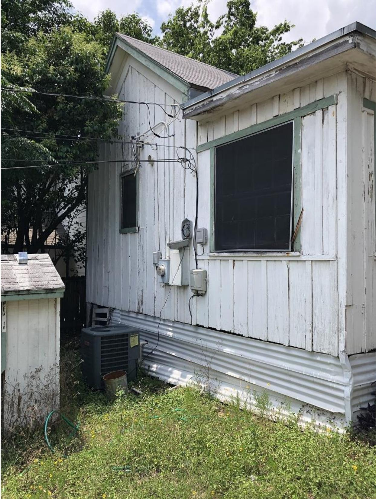
2. "Faux Victorian" Front windows are NOT original and not placement/locations are not consistent with period of significance-- replaced with mismatched sashes from other windows. These are windows are non-operable and screwed in place with pieces of filler wood and trim to fill in gaps.
