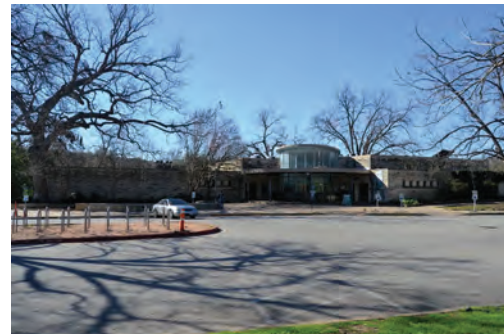
Zilker-Metro Barton Springs Bathhouse Rehabilitation
