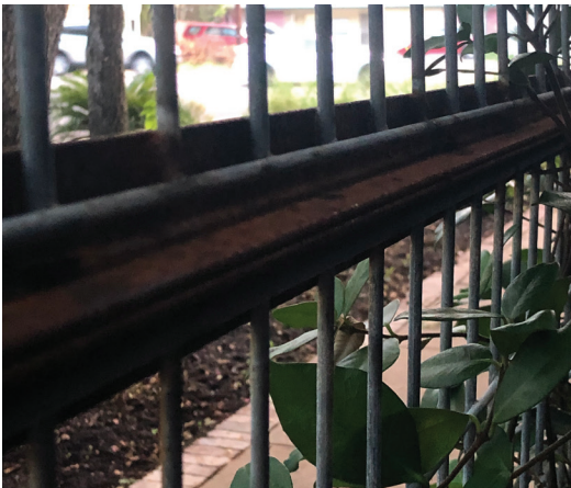
Wire panel welded to frame at mid-rail, property side facing
