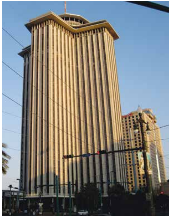
The World Trade Center of New Orleans, designed by Edward Durrell Stone, uses a simple bird-friendly strategy; almost all windows have exterior shutters. Photo by Christine Sheppard, ABC
