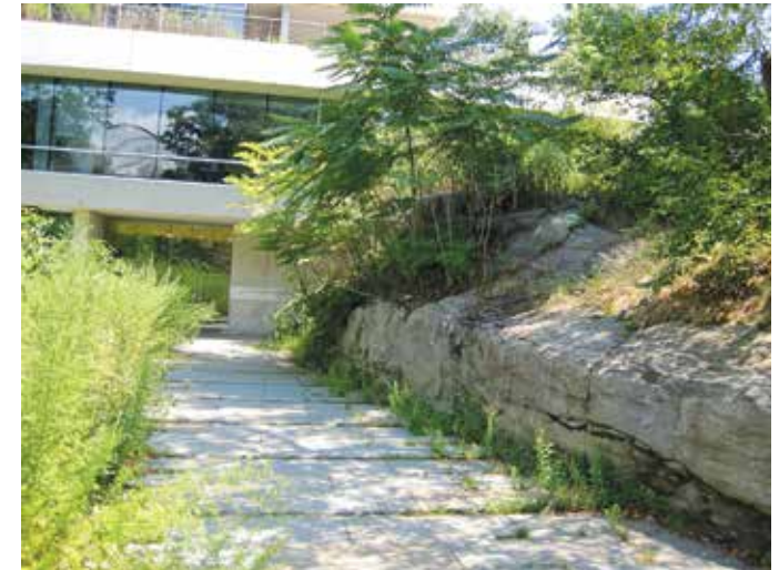
Birds flying from a meadow on the left are channeled toward the glass doors of this building by a rocky outcrop to the right of the path. Photo by Christine Sheppard, ABC
