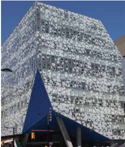
Snohetta's Student Learning Centre at Ryerson University is one of the first constructed under Toronto's design law. Photo by Rick Ligthelm
