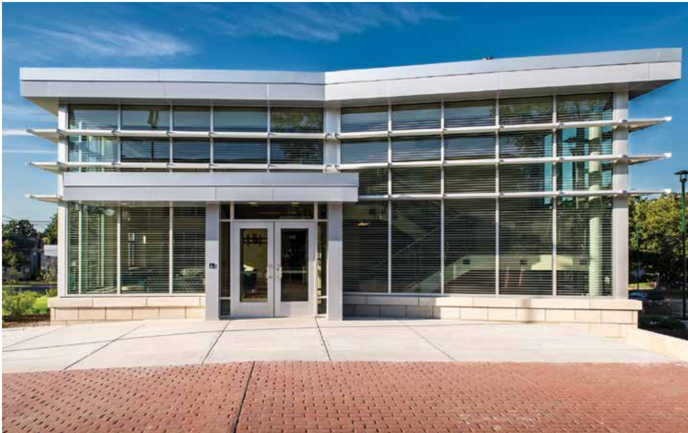
Use of glass with a highly effective horizontal frit pattern , together with sunshades, earned this retrofitted building on the SUNY Brockport campus the LEED “collision deterrence” credit. Photo by Paul Tankel
