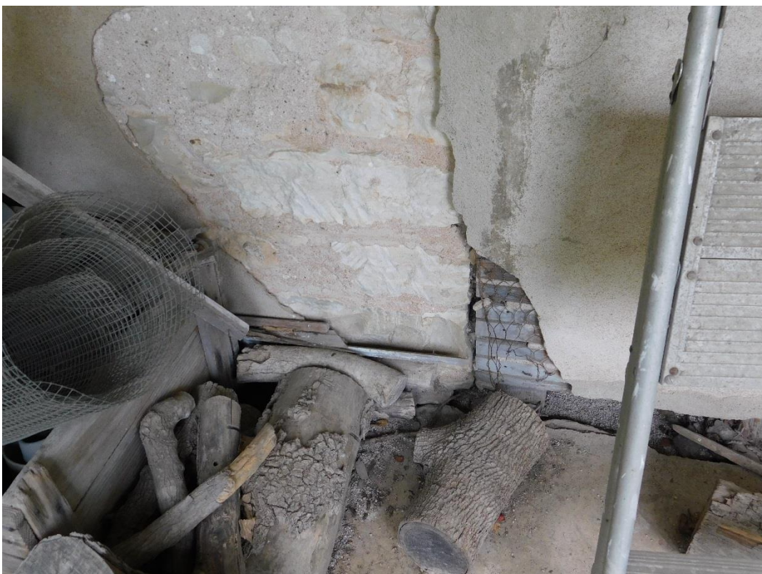
Photo showing the stone section (left) and the lathe section of the 1910s addition under the stucco on the east elevation of the house.
