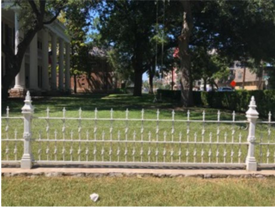
Existing fencing on south edge of the property. Fencing sits on a concrete footing. As the grade descends towards the west, the footing is faced with limestone rubble. This decorative mortar will not be necessary on the east façade, as the grade is relatively even and at its highest point on the east side of the property.
