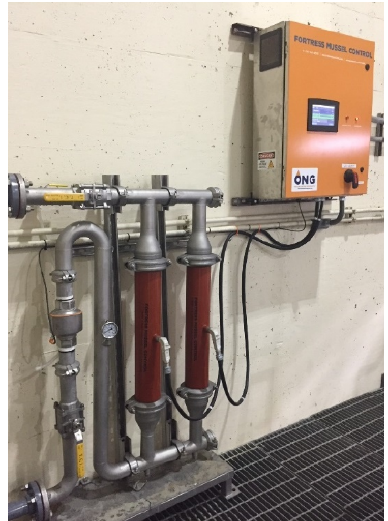
20 MGD Copper Ion Generator Lawrence, KS
