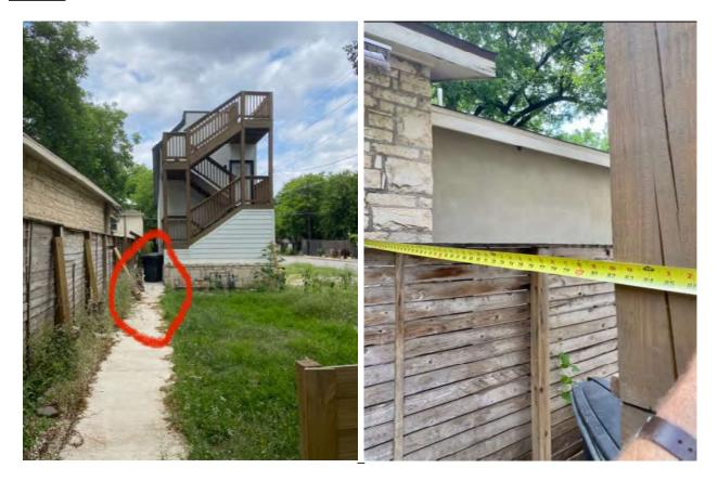
In practice, the as-built clearance is already quite tight and restricted. If the abutting property owner ever moves the fence to the property line—as is common during redevelopment activities—the sidewalk clearance will decrease from the existing 43" to a non-ADA—compliant width of 33" (2.78 feet).
