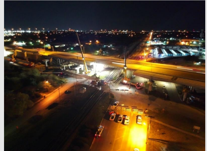
I-35 from US 79 to SH 45N (Northbound): Braided entrance and exit ramps beam set
