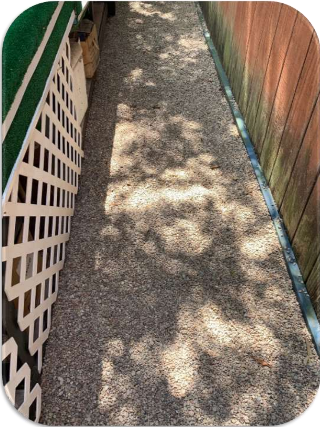
Area Between Pool and Former Workshop Showing Pavers Removed and Replaced with Pervious Cover
