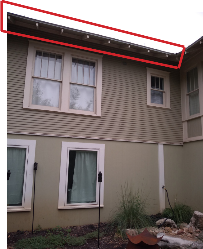
Partial south elevation portion of eave and roof to be demolished
