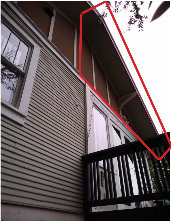
Partial west elevation (rear) portion of wall and roof to be demolished
