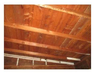
From the exterior of the addition we were able to observe that an elevated wooden floor framing system bears on a concrete slab. The photograph at lower left documents this framing pattern, as well as the deterioration of the sole plate for the exterior wall. The photograph at lower right is in the same general area, but a broader perspective. This photograph indicates that the water damage (rot) continues up the wall to the siding and presumably to the wall framing.
