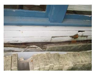
For this type of wall construction the building code (International Residential Code) requires a minimum of six inches from grade to the top of the foundation to prevent surface water intrusion. This clearance was not provided. The result is extensive deterioration of the exterior wooden framing.
