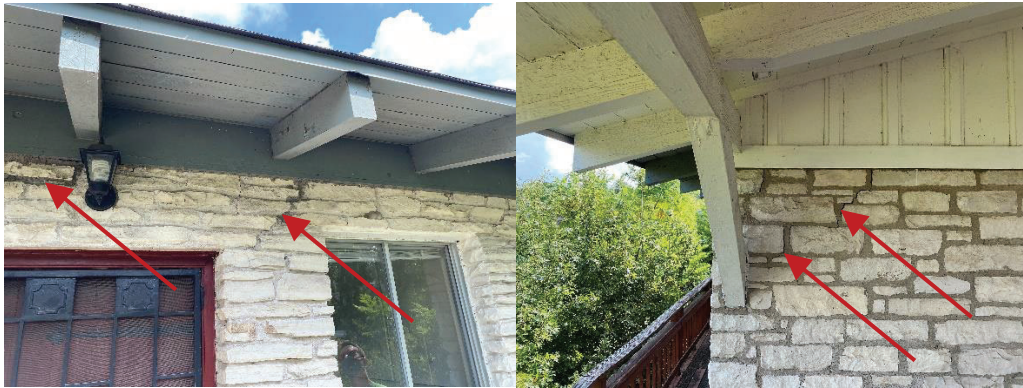
Figure 5. Cracks in stove veneer.
