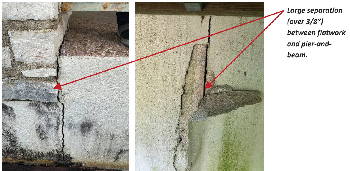
Figure 4. Dissimilar foundation types
