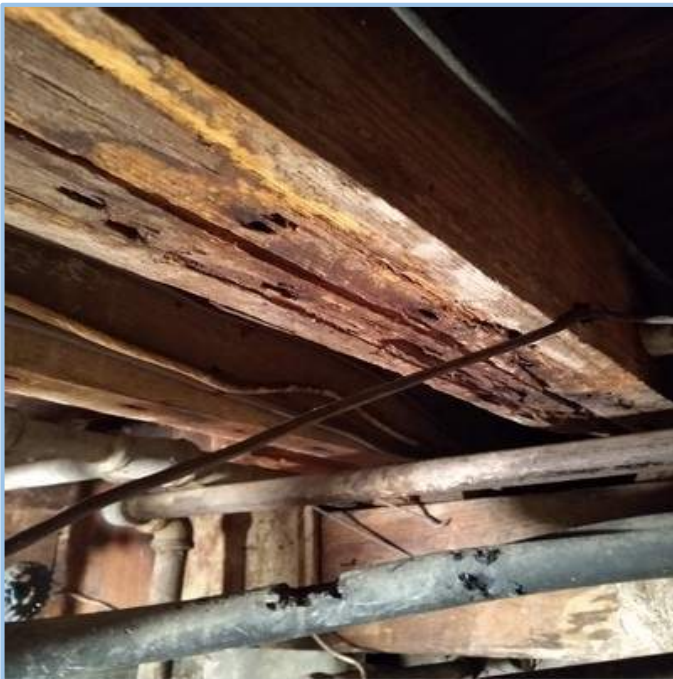
Severely Rotted Wood Joist Framing at Crawlspace
