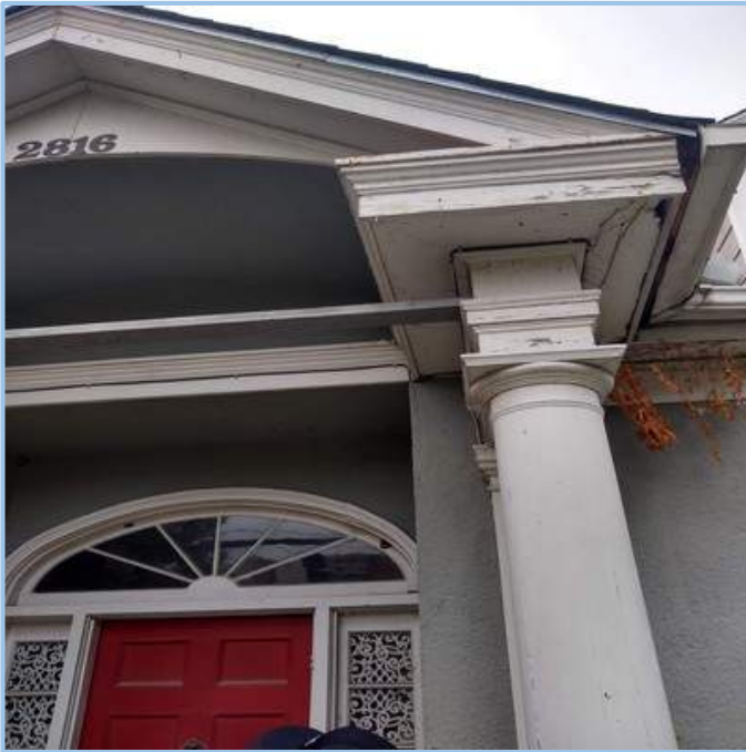
Rotted Wood at Building Facade
