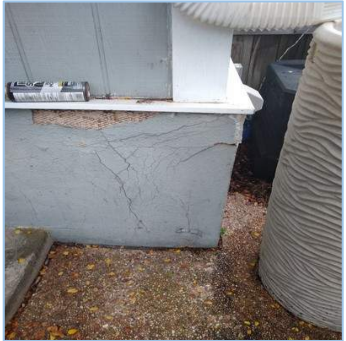
Stucco Cracking at Building Skirt
