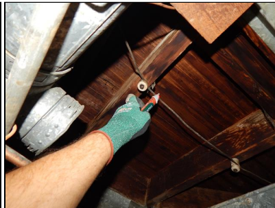
Spliced knob and tube wiring.
