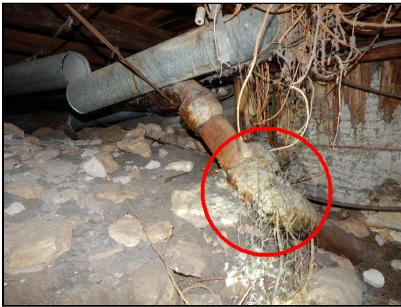
Pipe attachment failed.
