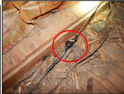
Spliced knob and tube wiring.
