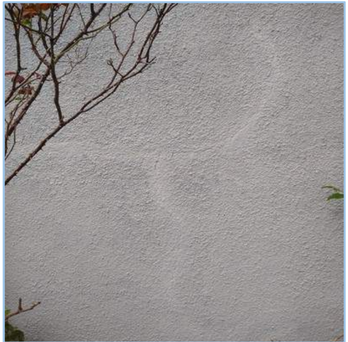
Evidence of Prior Stucco Repairs
