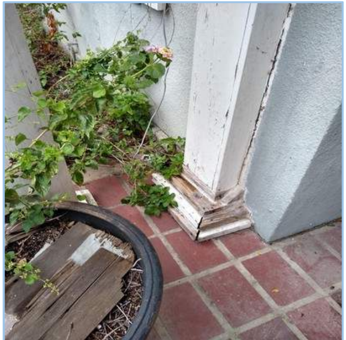
Deteriorated Wood at Base of Column
