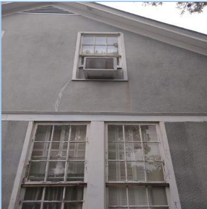
Diagonal Crack at Window Opening
