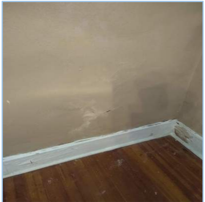
Evidence of Water Infiltration at Exterior Wall
