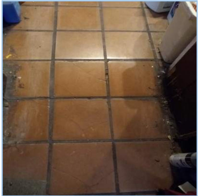
Bulging Tile at Rear Addition Due to Foundation Movement
