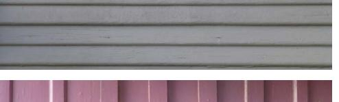
Wood is the most common type of siding in Austin, as it was easily milled into different shapes, with profiles that changed along with architectural styles.
