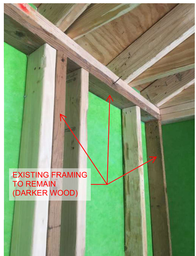
Garage photos showing original framing, and relationship to property line.
