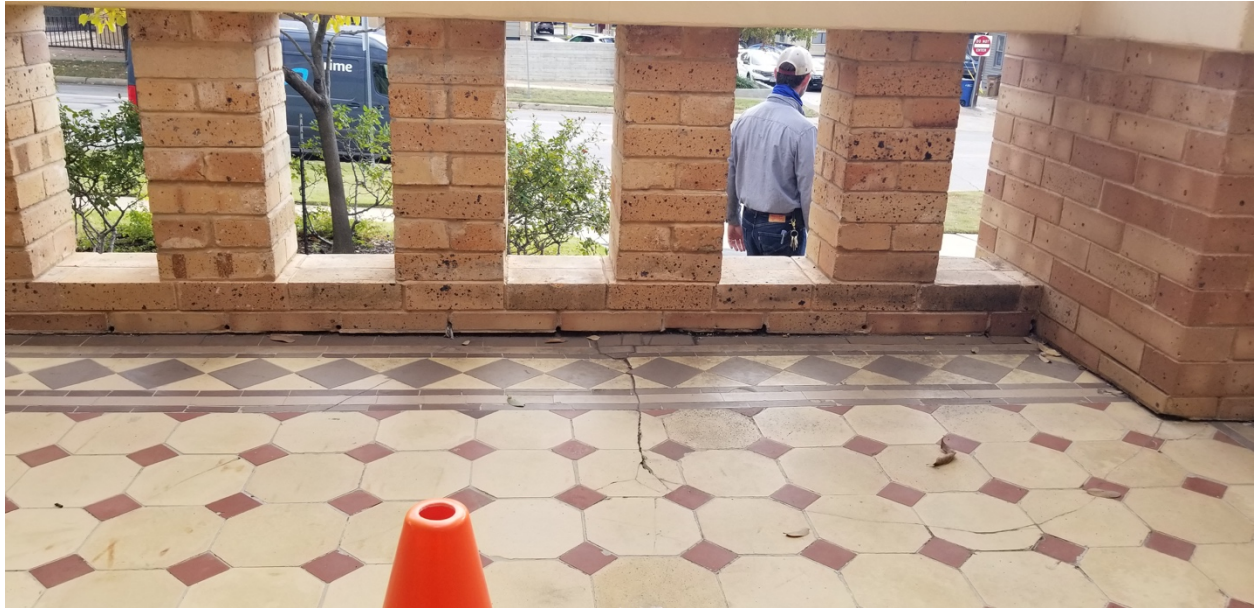
Detail at east side of the southeast corner of first floor porch showing original encaustic tiles and evidence of displacement, November 2020.
