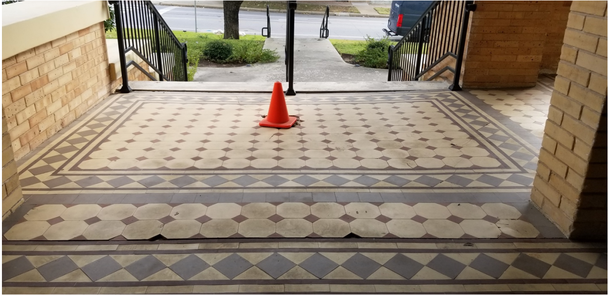
Original encaustic tiles and evidence of displacement at the northeast corner of the first floor porch, November 2020.
