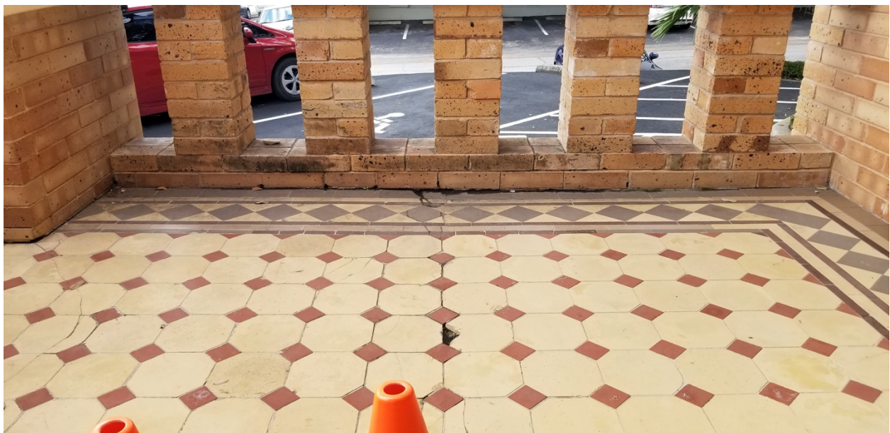
Detail at south side of the southeast corner of first floor porch showing original encaustic tiles and evidence of displacement, November 2020.
