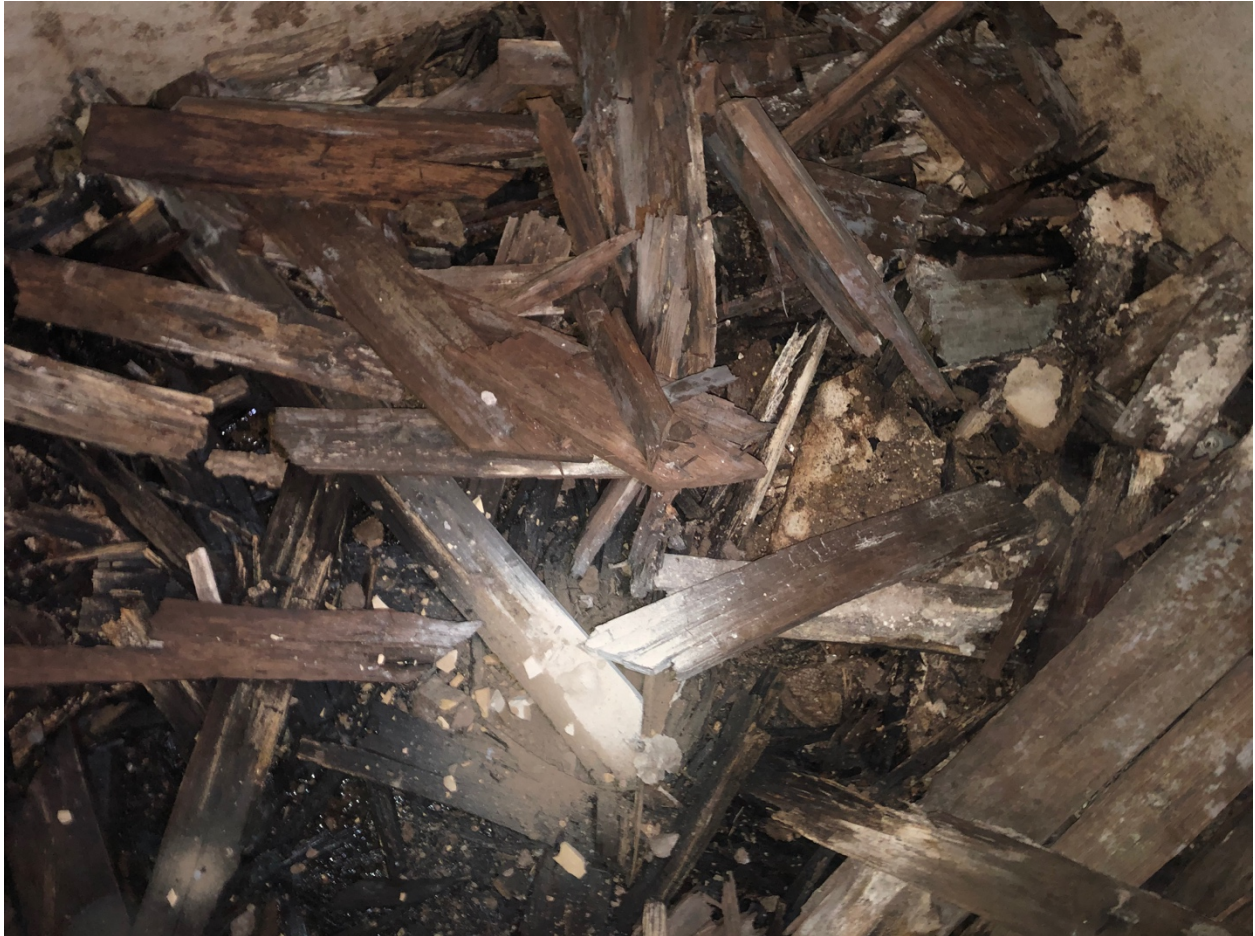
Photo of collapsed floor joists in the cavity below the southeast corner of the first floor porch, July 2020.
