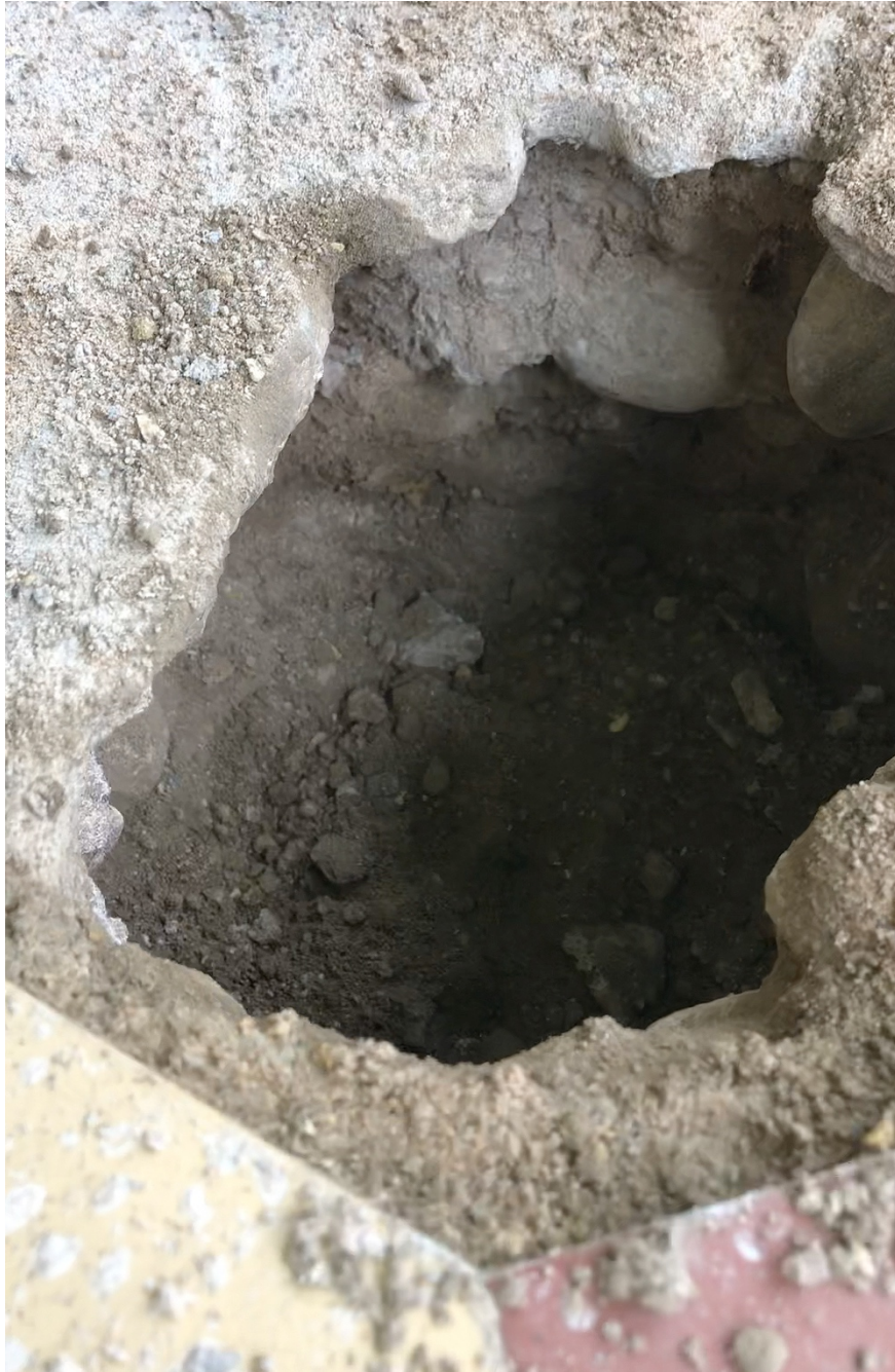
Photo of dirt and gravel base directly below historic porch slab at the northeast corner of the first floor porch, July 2020.
