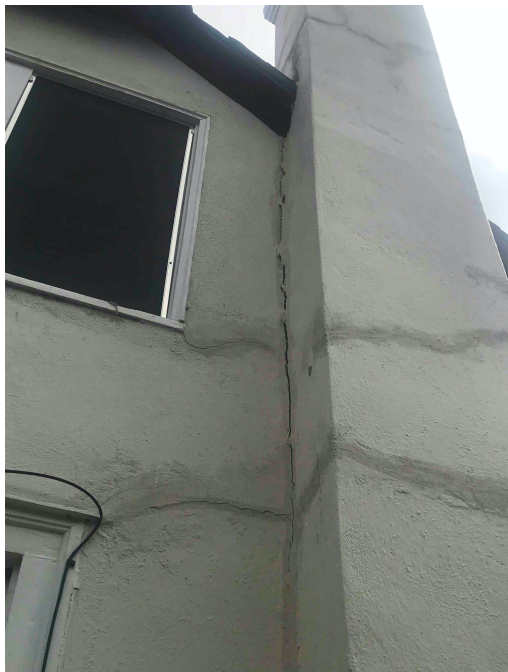
Cracks from shifting foundation
