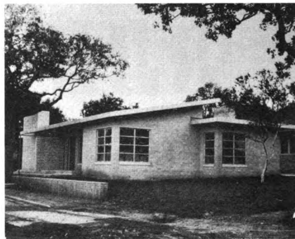
FIG. 5--Building No. 4. Walls are of solid tile; roof is a single sloping joistile slab.
