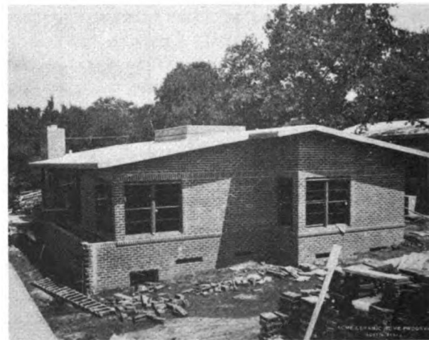
FIG. 7--Building No. 3. Walls are 10-inch cavity type, of dense brick and dense tile.
