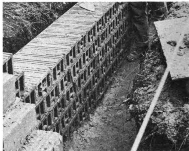
FIG. 3--A section of tile foundation for one of the all-ceramic residences.
