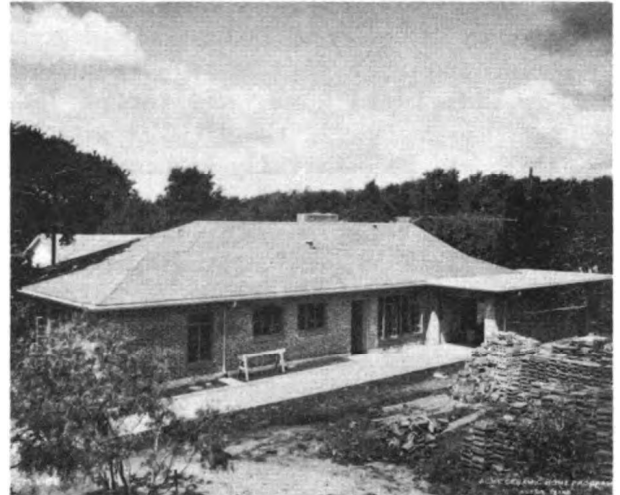
FIG. 9--Building No. 1. Walls are 10-inch cavity type, of soft brick and soft tile.
