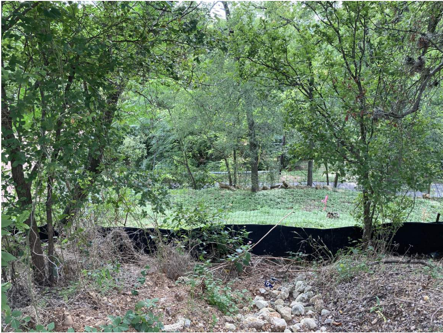
11. Silt fence at undeveloped alley portion
