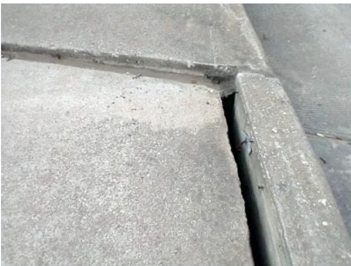
Bridge cracks are large enough to catch bicycle tires which increases the likelihood for accidents and propelling riders into Slaughter traffic.
