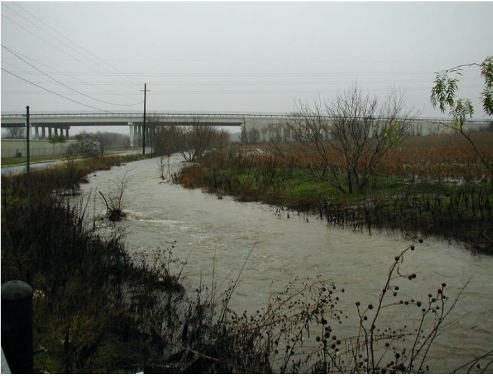
Flooding along eastern edge of subject track. This stormwater flows into the detention pond at the Hollows at Slaughter Creek and often carries flood debris causing potential blockage. Slaughter Creek drive is impassable during large storm events.
