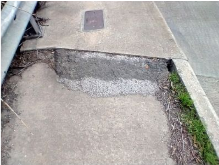
Bridge is separating from sidewalk causing pedestrian and bicycle safety concerns. Repairs are failing.
