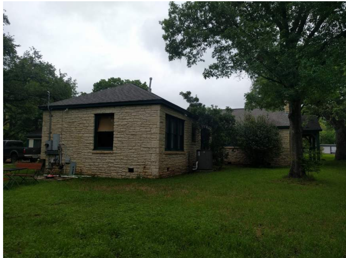
Existing Rear Elevation, Looking East
