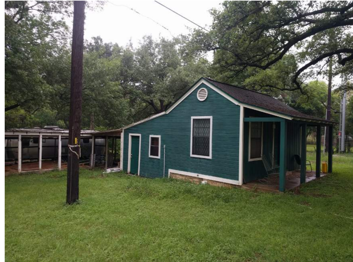
Existing Guest House, Looking West (No Work)
