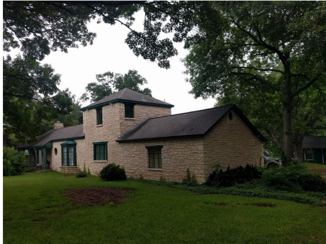
Existing Front Elevation, Looking South West
