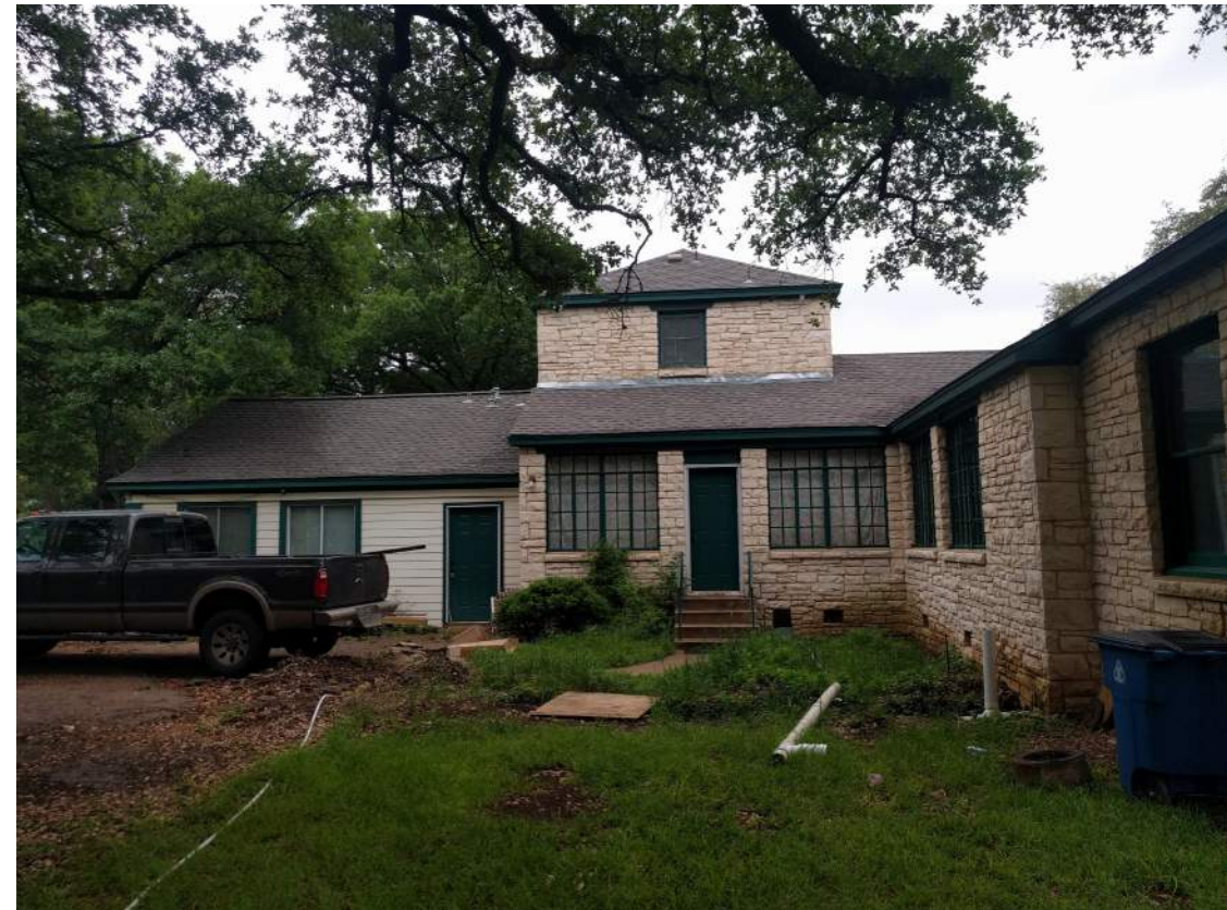
Existing Rear Elevation, Looking East
