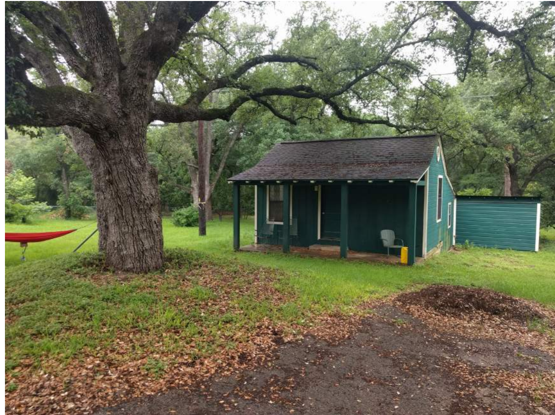
Existing Guest House, Looking East (No Work)
