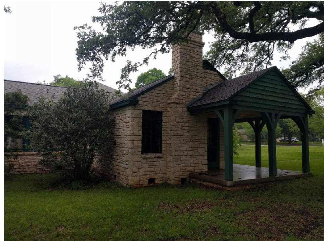
Existing Elevation, Looking North East
