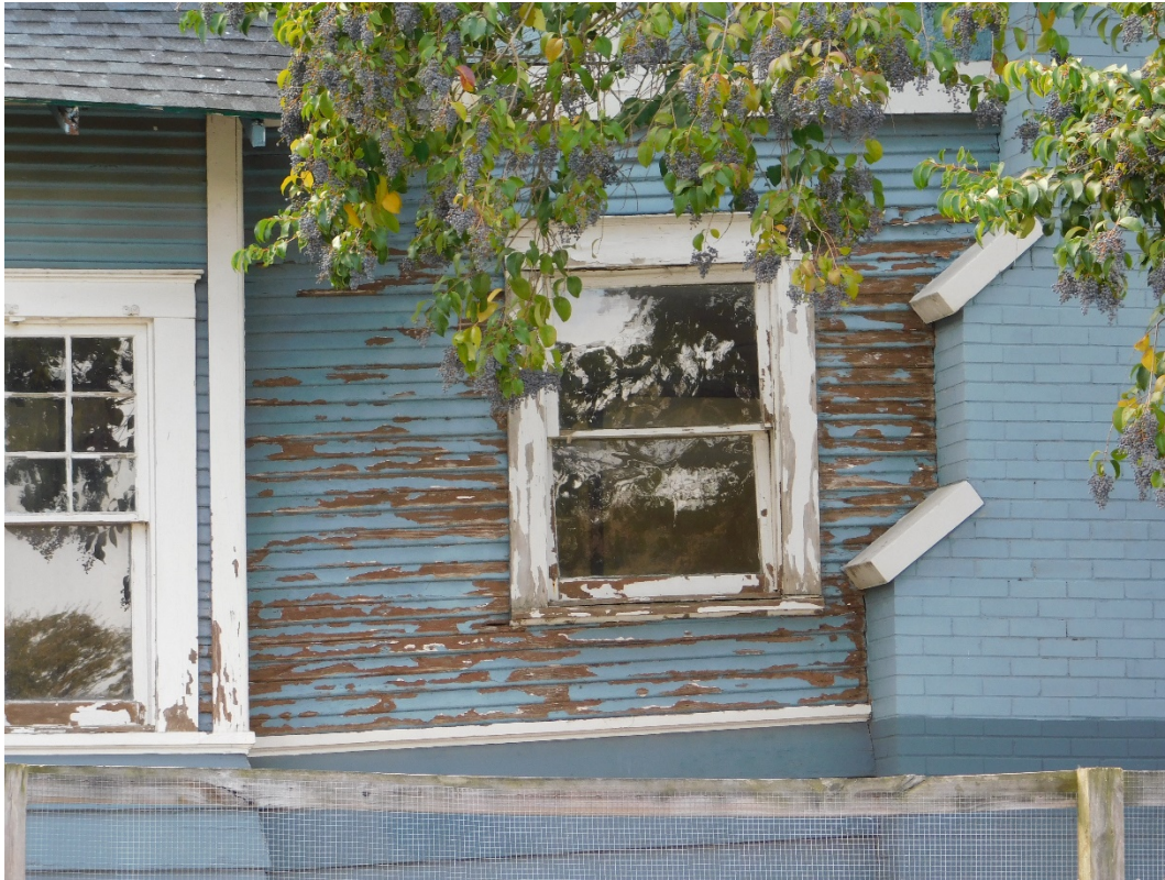
Photograph showing the north side of the house where the foundation has failed; the window has sagged, and much of the wood siding and window frames exhibit extensive rotting.
