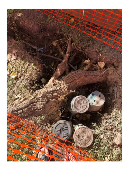
Root was excavated by Austin Water – Roots are clearly destroying pipes.
