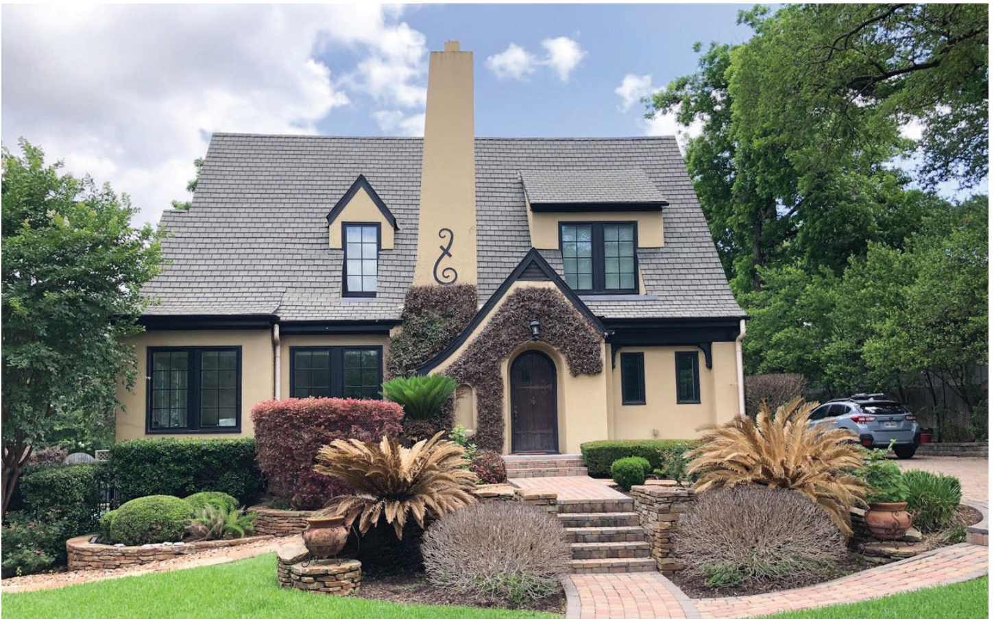
Original windows on the south façade included multi-light casement and 1:1 windows on the first floor and 6:6 double-hung sash in the dormers. Google Street View, March 2011.
