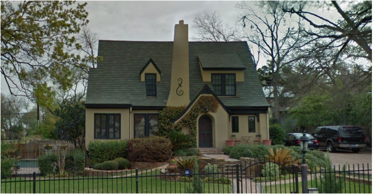
Original windows on the south façade included multi-light casement and 1:1 windows on the first floor and 6:6 double-hung sash in the dormers. Google Street View, March 2011.
