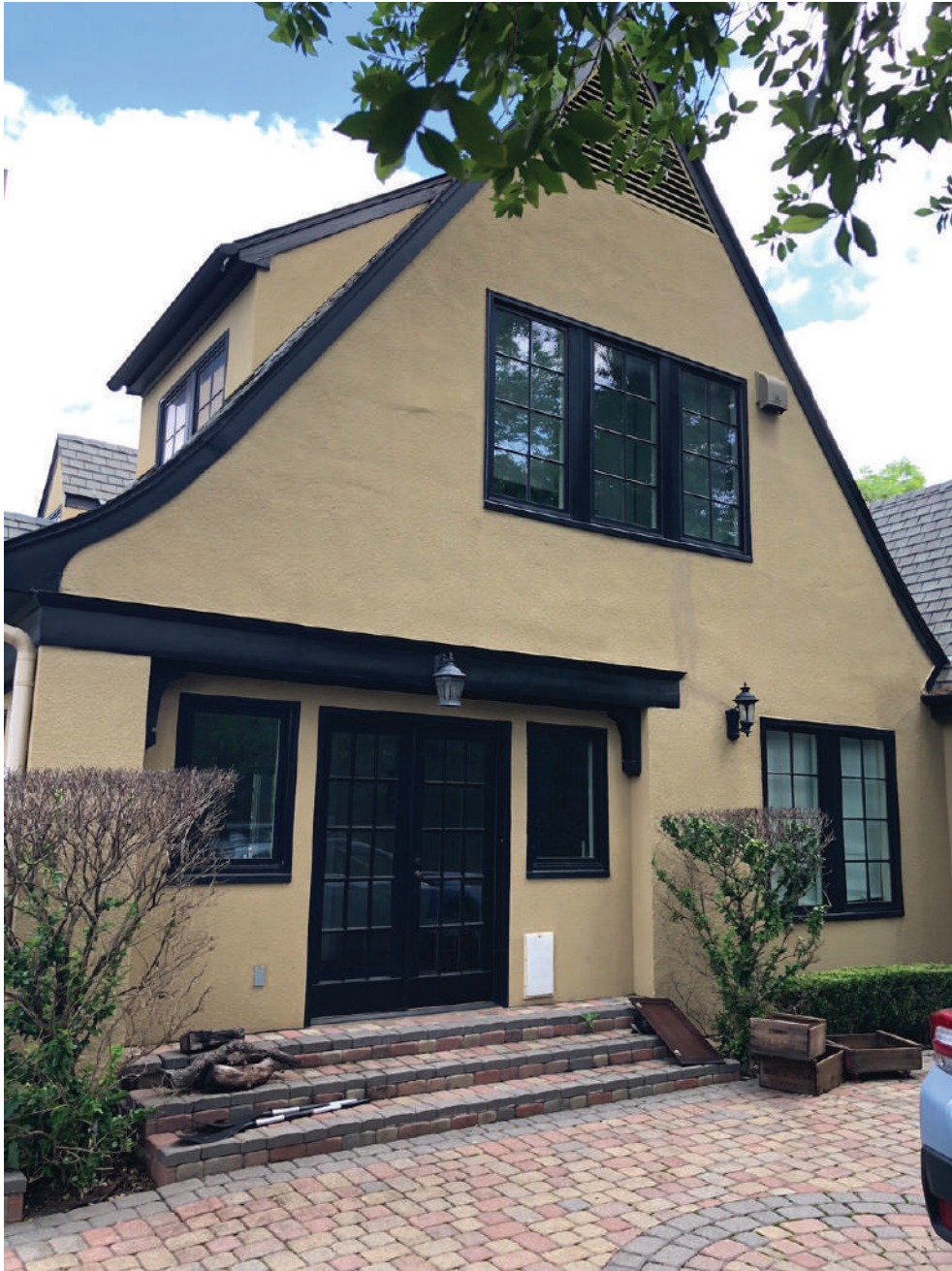
SIDE ENTRY DOORS AND WINDOWS TO BE REPLACED WITH NEW DOOR AND WINDOW IN MATCHING STYLE OF EXISTING HOUSE. REAR ENTRY DOORS TO BE REPLACED WITH NEW WINDOW. (WINDOWS AND DOORS PROPOSED TO BE REPLACED ARE NOT ORIGINAL TO THE HOUSE.)
