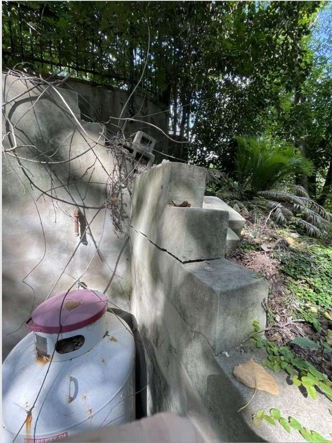
3401 RIVERCREST - FAILING RETAINING WALL DETAIL
