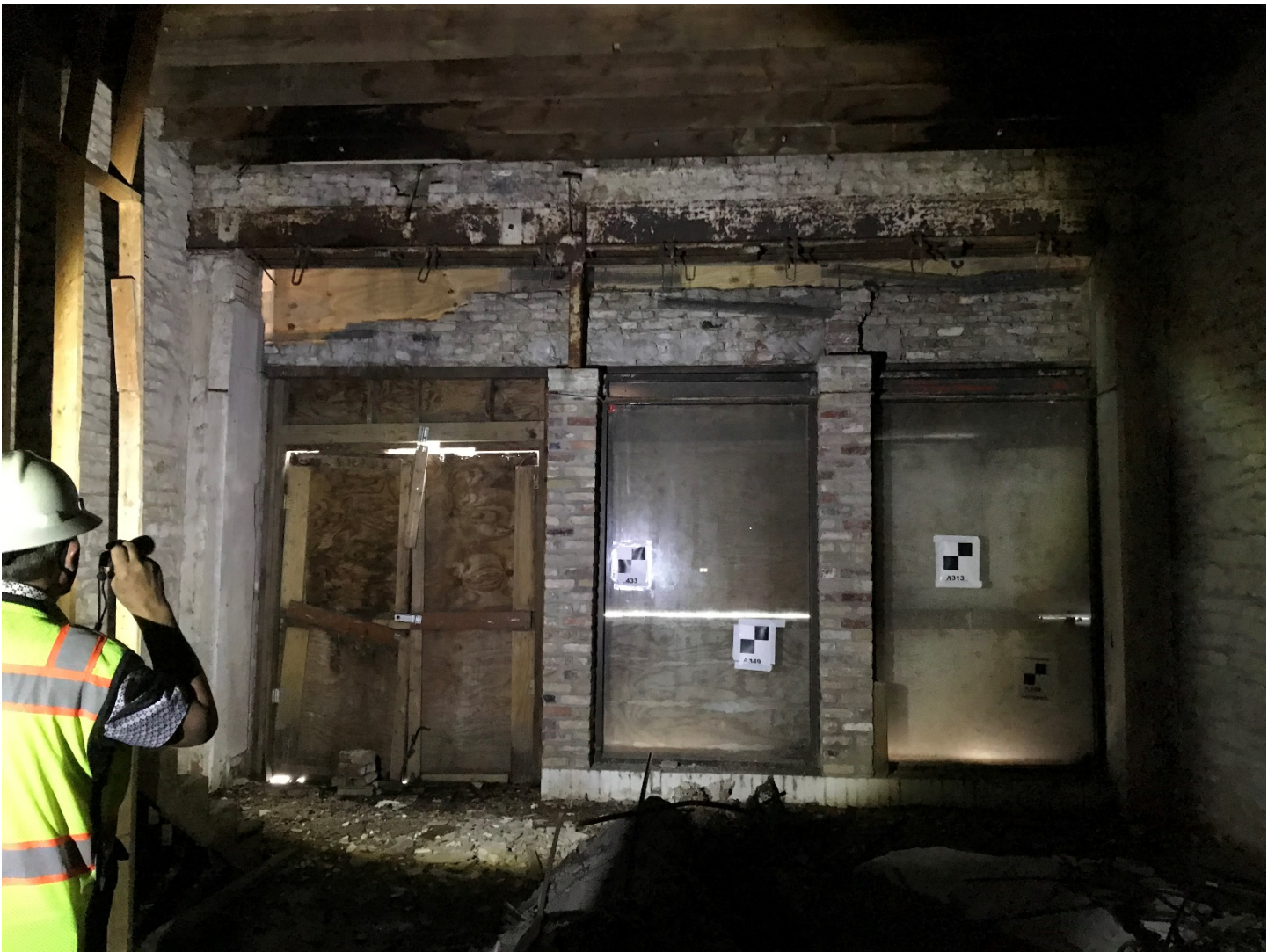
Interior of 911 Congress Ave. storefront, Historic Preservation Office staff, May 2021. Note added steel beam and failing brick storefront.
