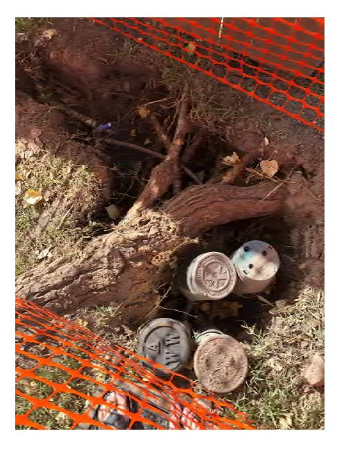
Root was excavated by Austin Water – Roots are clearly destroying pipes. 52 of 73
