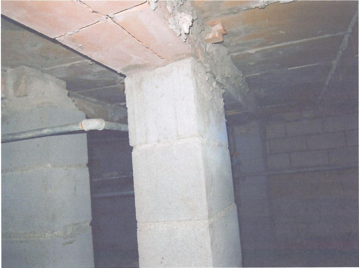
**Another photograph of supporting masonry column believed to have been installed prior to 1959 under floor of room on west side of garage**
