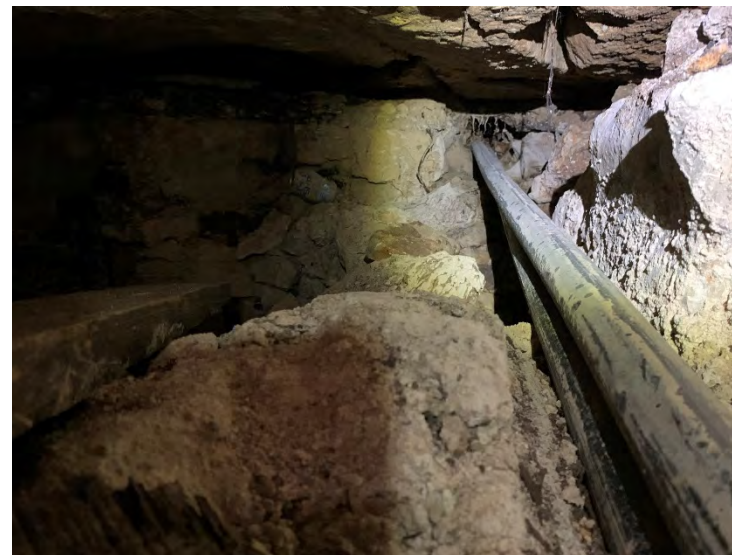
PHOTO 8 View of 2-inch-diameter buried steel piping running through cave next to WWL, facing north
