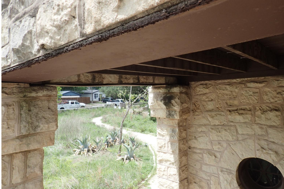
Photo E: Existing Steel Lintel
