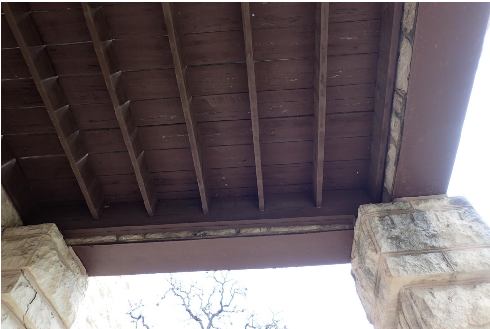
Photo D: Balcony Wood Framing
