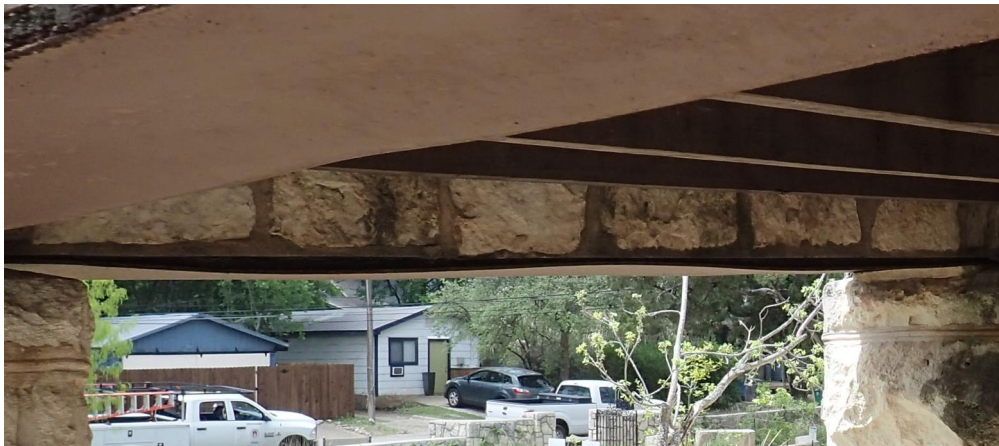
Photo F: Existing Steel Lintel
