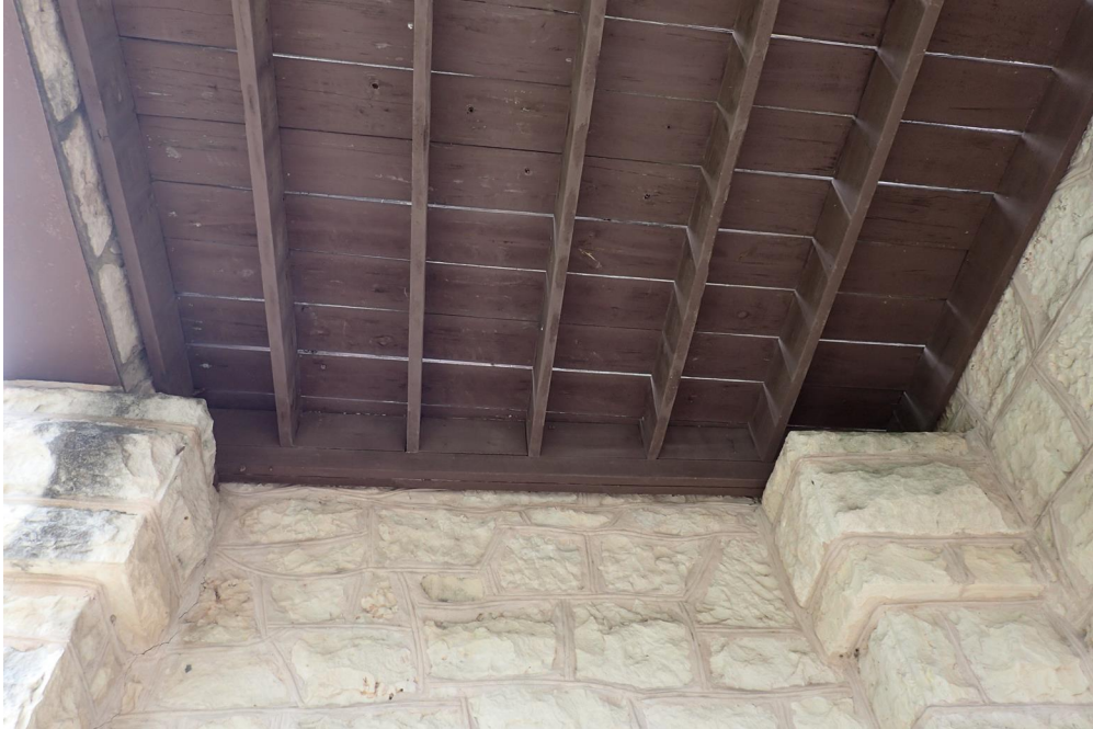
Photo C: Balcony Wood Framing
