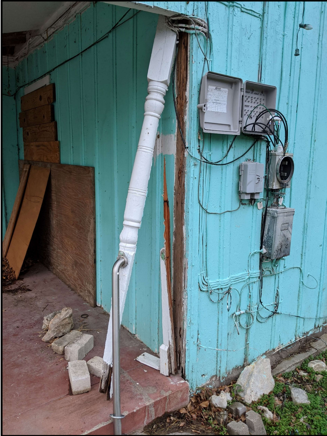
Figure 4.12: Close up view of engaged column at north end of porch and existing electrical, telephone, and cable television utility services.
