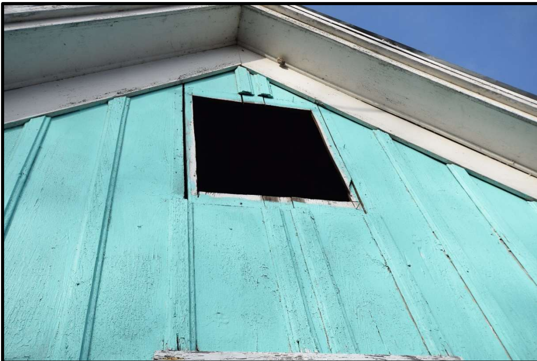
Figure 4.25: Close up view of missing vent at east gable end.
