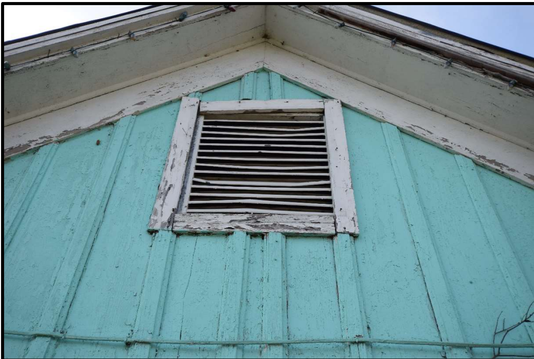
Figure 4.14: Close up view of painted metal louvered vent at gable end of front wing.
