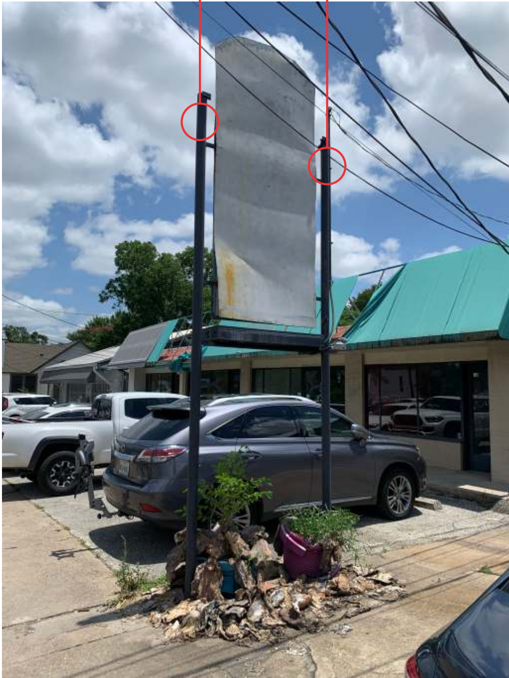
Existing double-pole setup to be re-used
