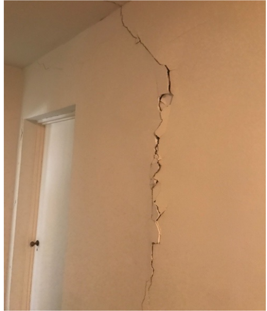
Figure 2 – Cracks in Plaster
