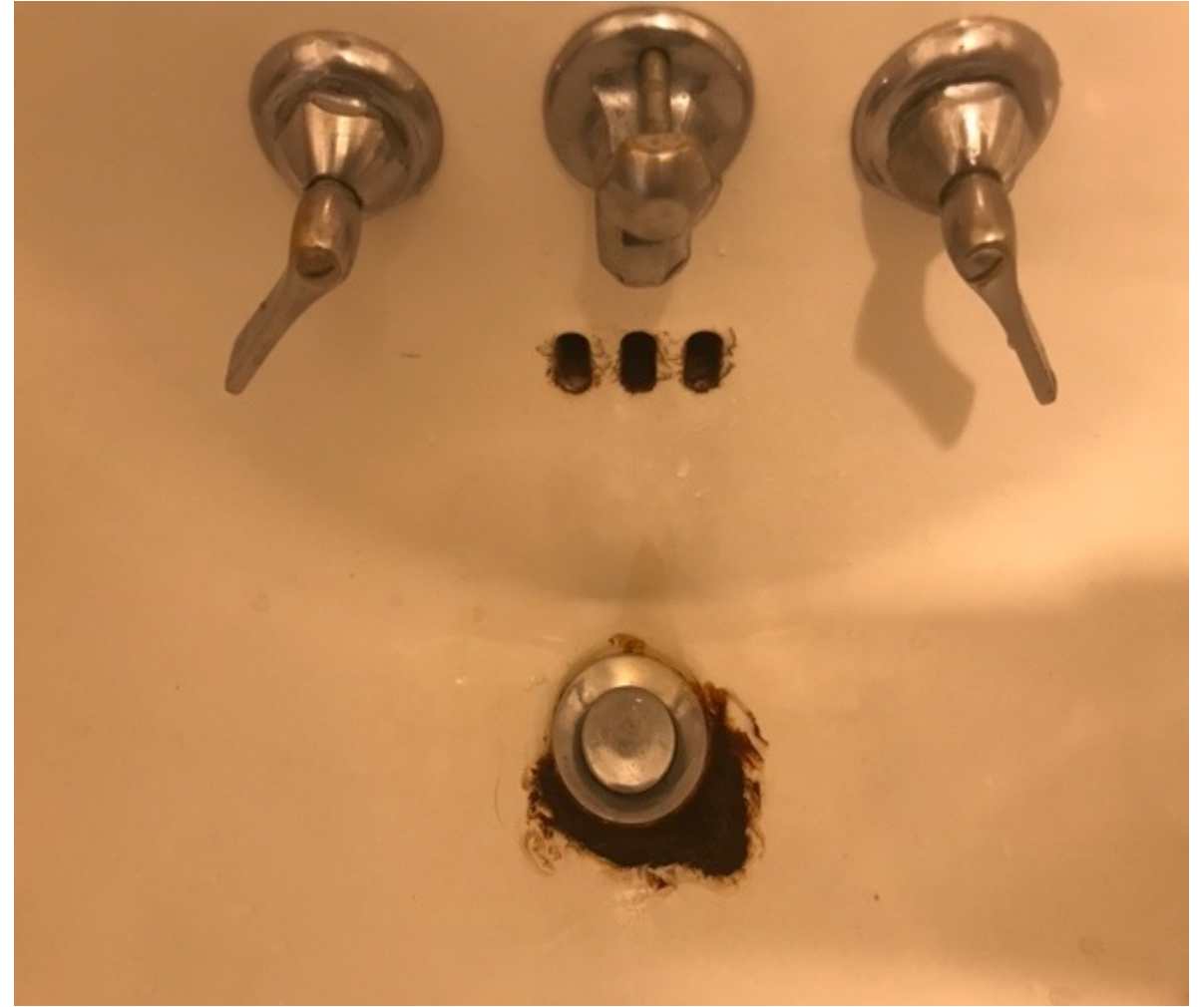
Figure 10 – Antiquated Plumbing Causing Water Pressure and Clog Issues
