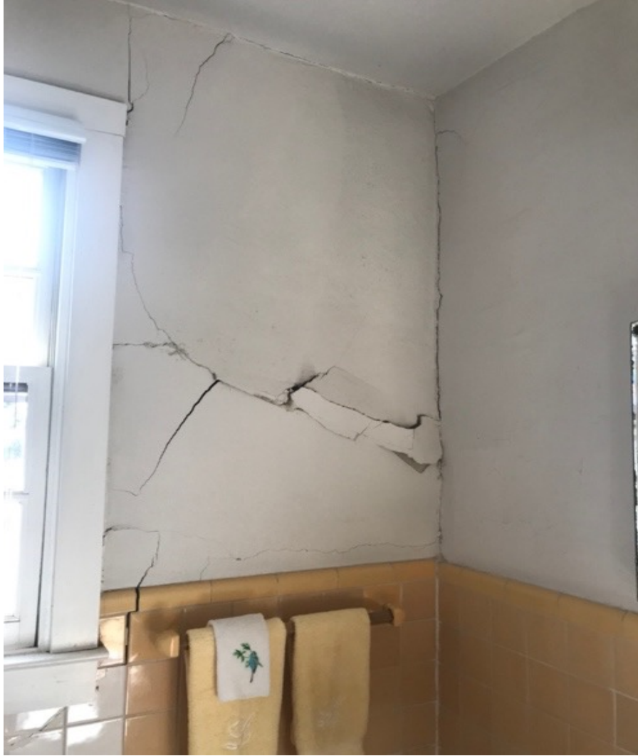
Figure 1 – Cracks in Plaster
