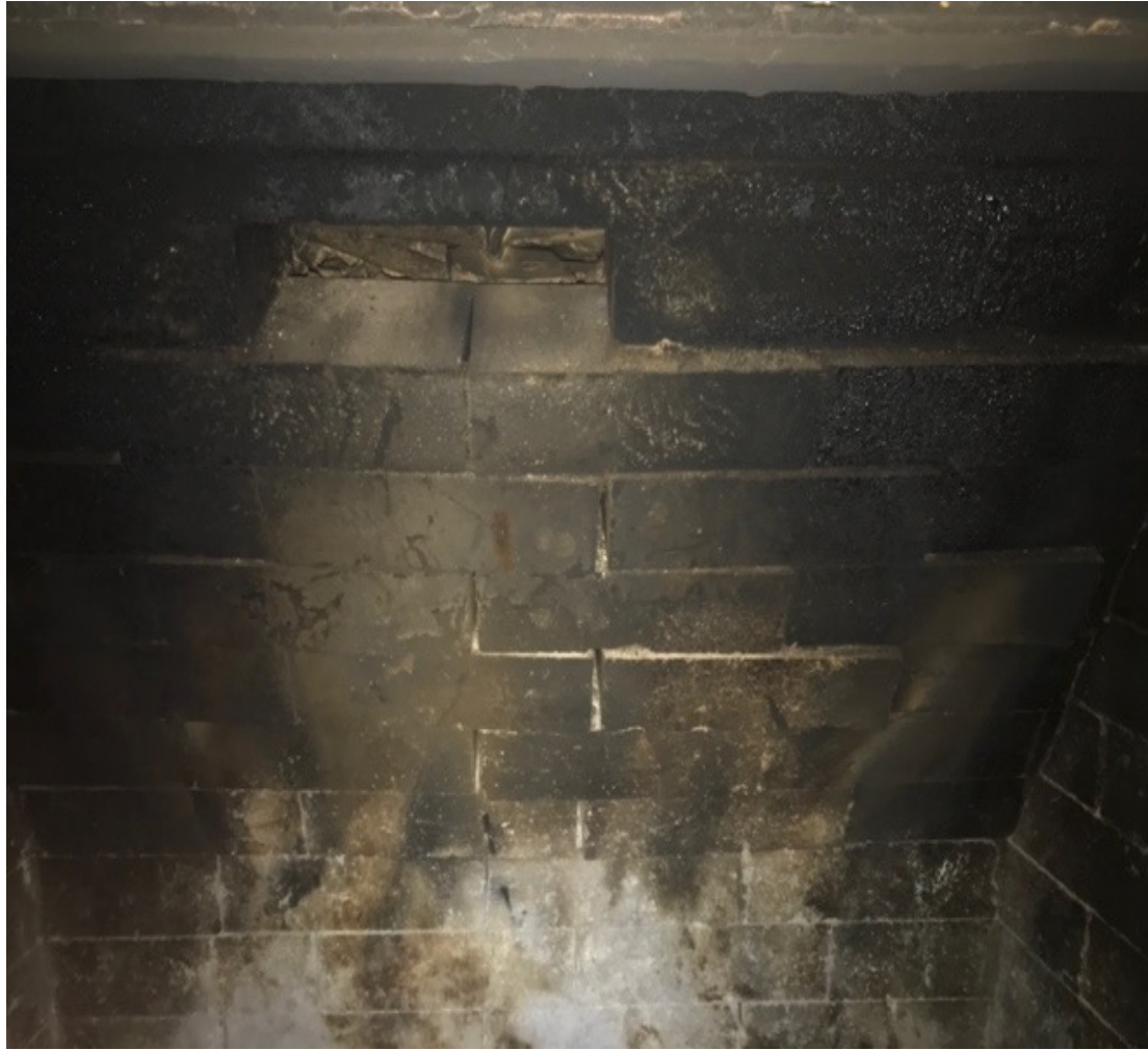
Figure 9 – Fireplace with Deteriorating Brick Liner and Heavy Creosote
