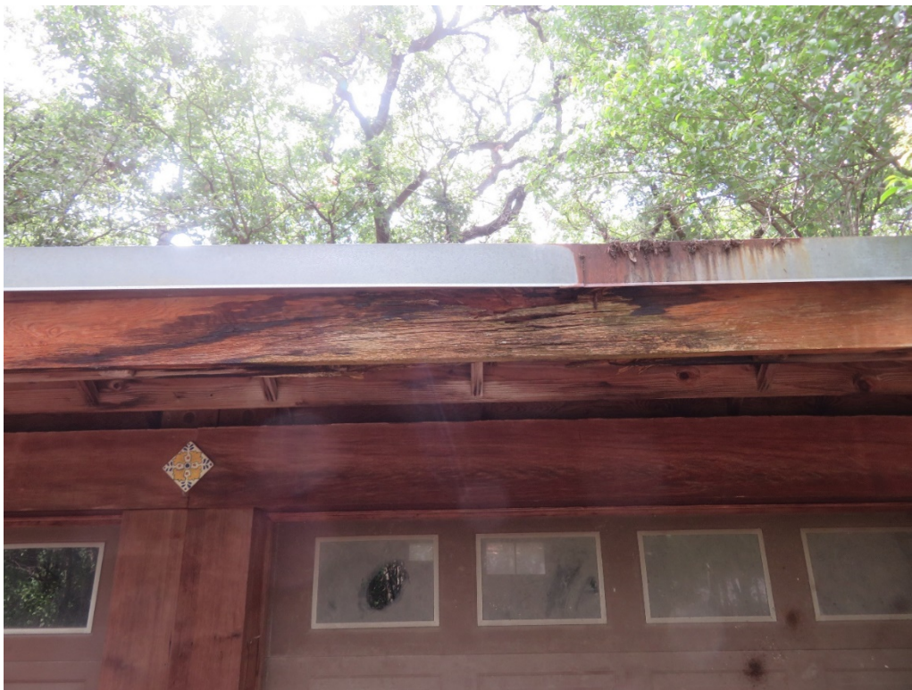
Detached garage water damage of main support cross beam.
