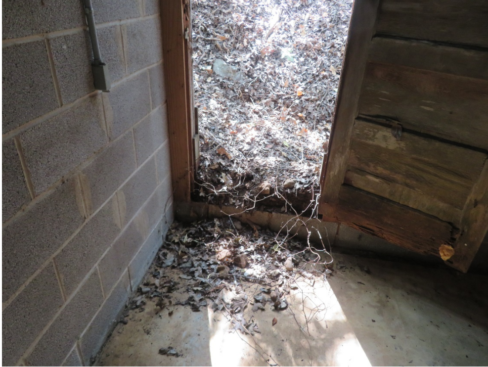
Extensive erosion into detached garage due to lack of landscaping.
