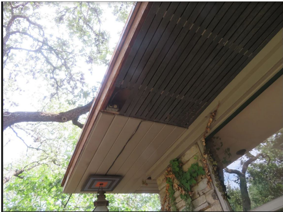
Self-installed lighting, code violation
