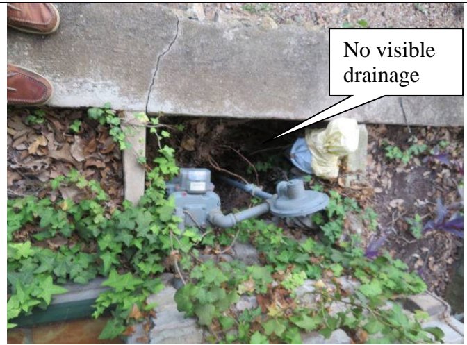
42. Gas meter pit (looking down)
