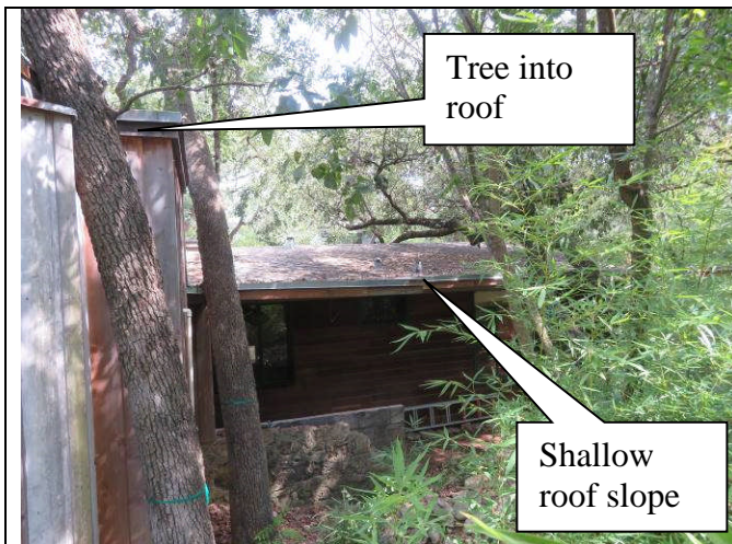
33. Shallow pitch roof at rear
