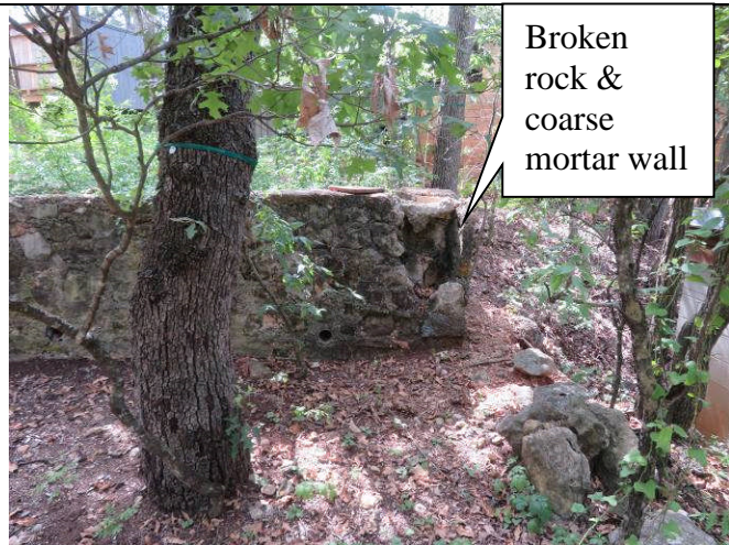
11. Typical stone rubble wall construction
