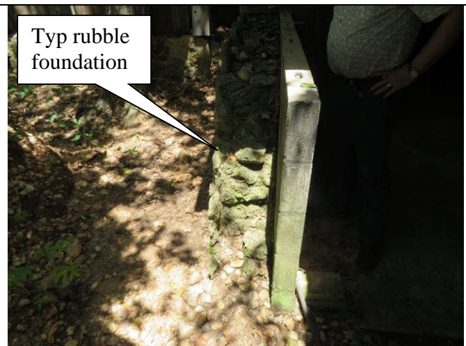
34. Typ rubble filled foundation wall
