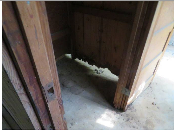
9. Rotted garage walls - typical
