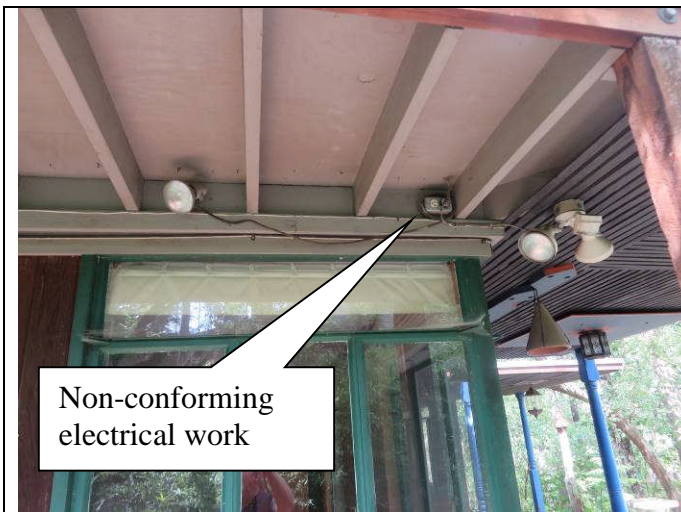
45. DIY electrical wiring and fixtures
