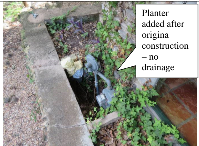
12. Gas meter at original grade
