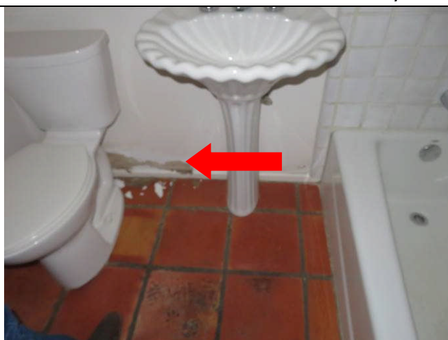
68. Water damage at bathroom ext'r wall
