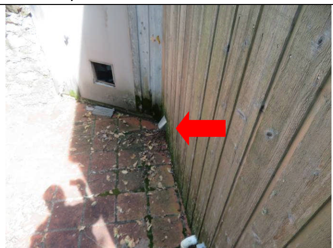
38. Rot / leaks at utility room wall base
