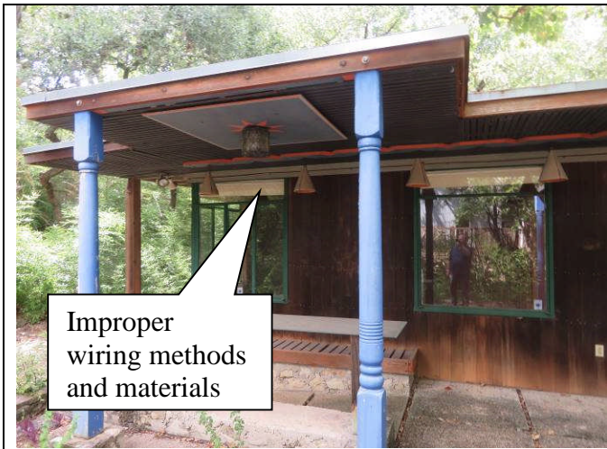
57. Light fixtures not rated for outdoor use
