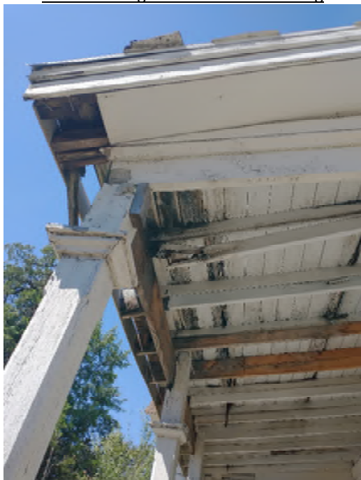
Rotted and Damaged Roof Framing
