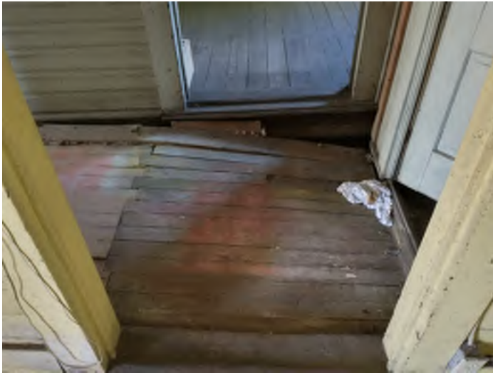
High Levels of Foundation Movement
