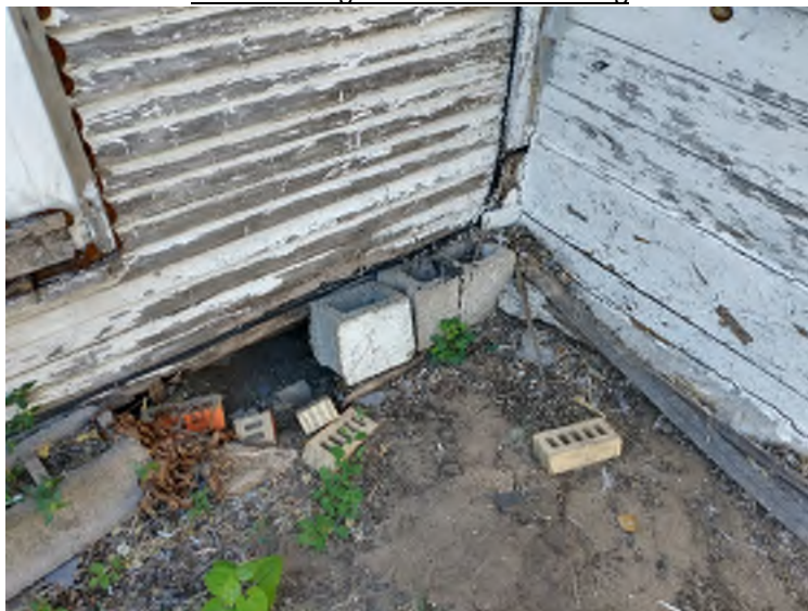
Water Damaged Studs and Sheathing
