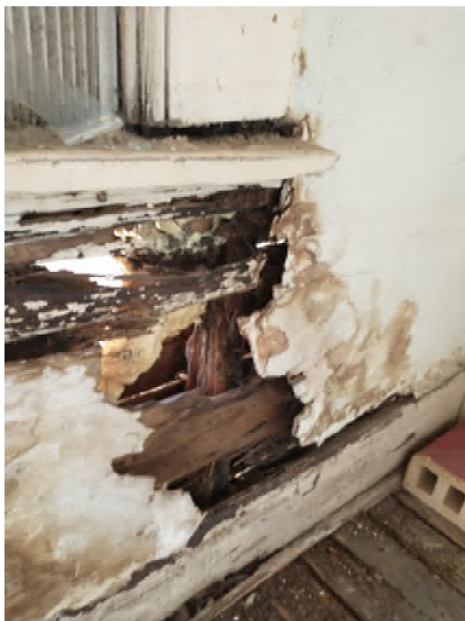
Water Damaged Studs and Sheathing
