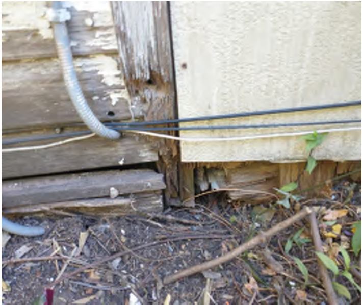
Rotted Wood in Contact with Ground
