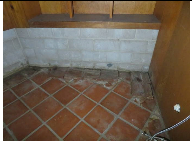
66. Water leaks at exterior wall - utility
