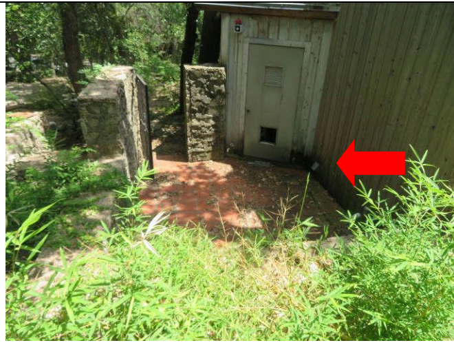
39. Rot / leaks at water heater closet
