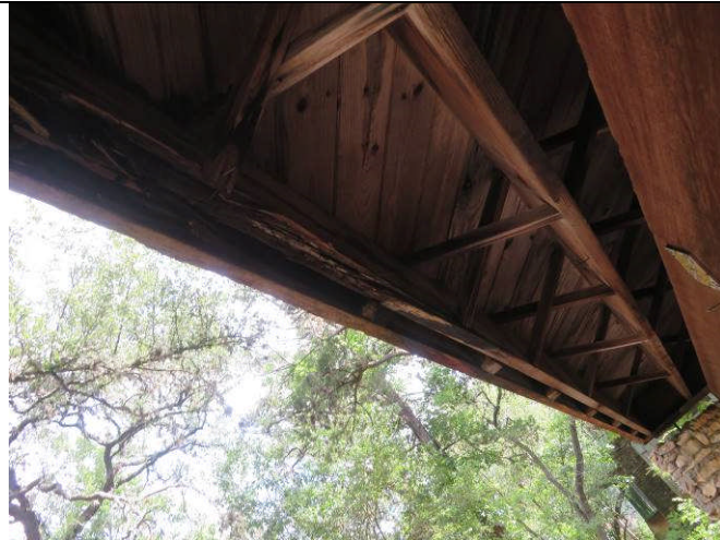
5. Rot under garage roof overhang
