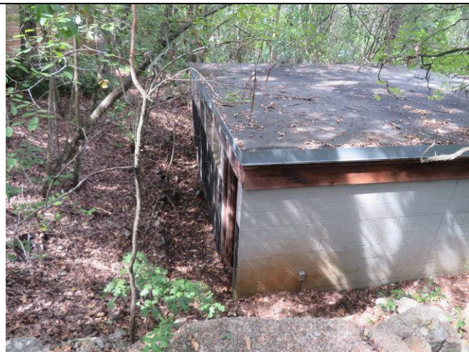
7. Soil above garage floor grade on 3 sides
