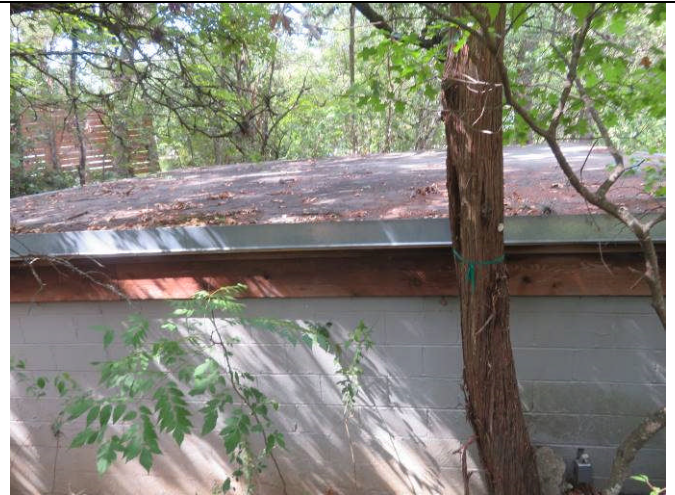
6. Garge roof ponds water
