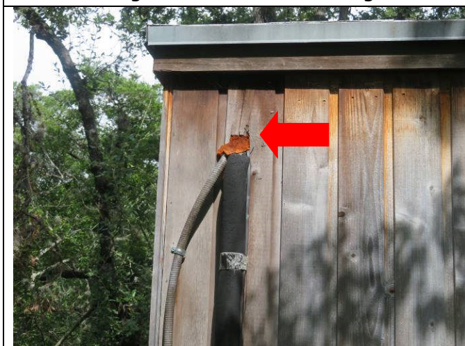
37. No flashing at wall penetration
