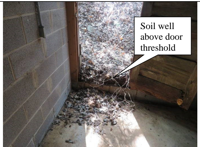
8. Soil above garage floor / water leaks
