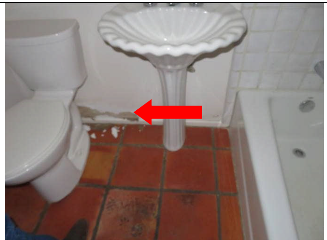
68. Water damage at bathroom ext'r wall
