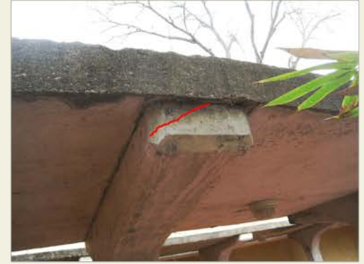
C SHELTER REPAIR x2 = 1/2"
