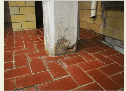
F SHELTER REPAIR x2 = 1/2"
