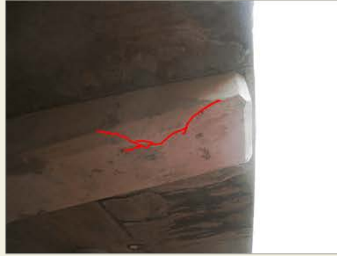
B SHELTER REPAIR x2 = 1/2"
