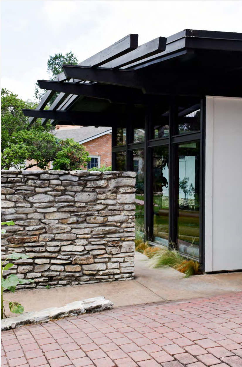
Photo 5. Detail of projecting front ell, carved roof joists, and pergola of open rafters; oblique view inside garden wall, camera facing south-southwest, Rubinett House, 3004 Belmont Circle. Photo by HHM, May 2021.
